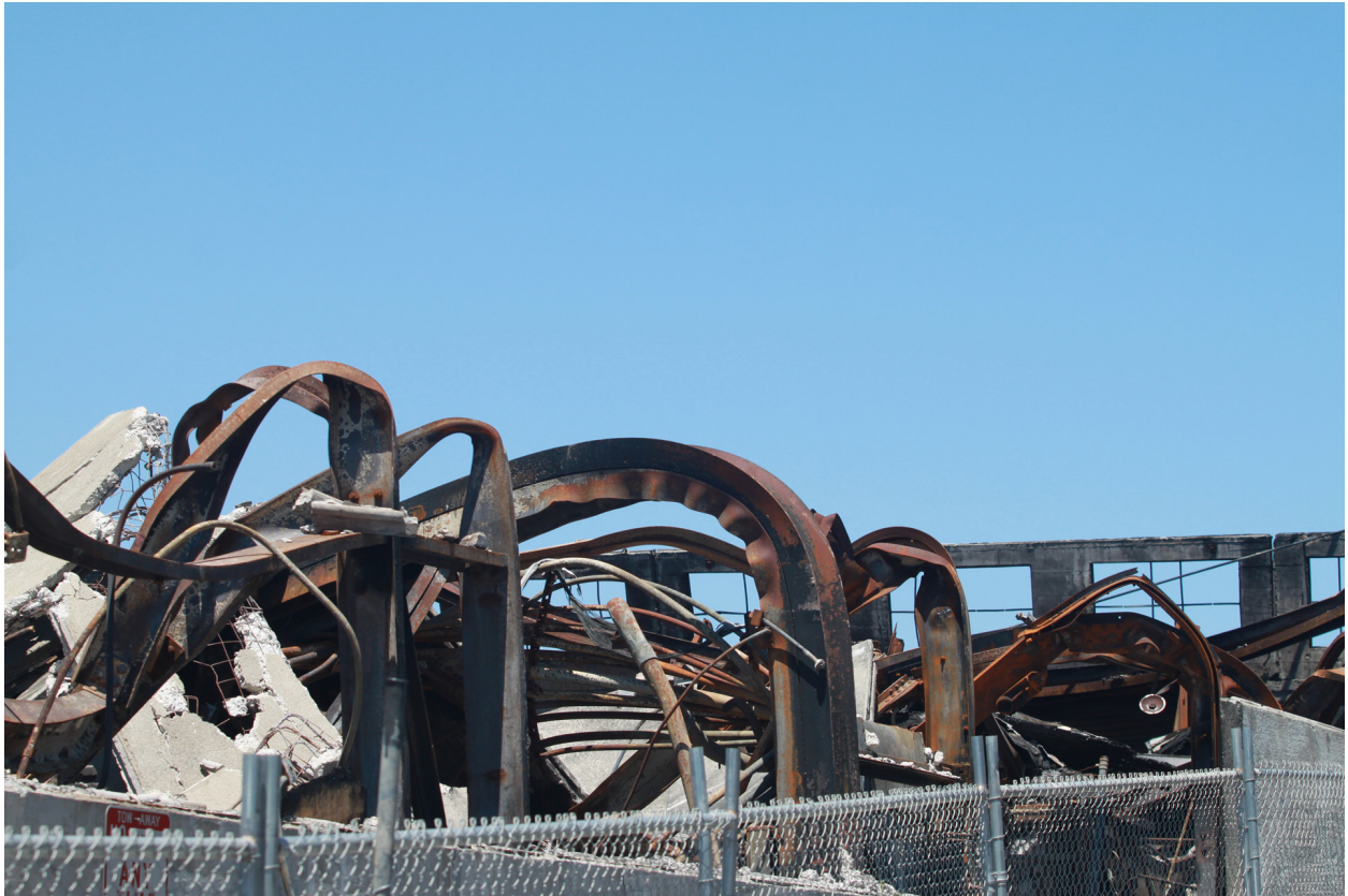
Figure A.20: Bending of column in the weak axis direction, with local buckling in flanges.
