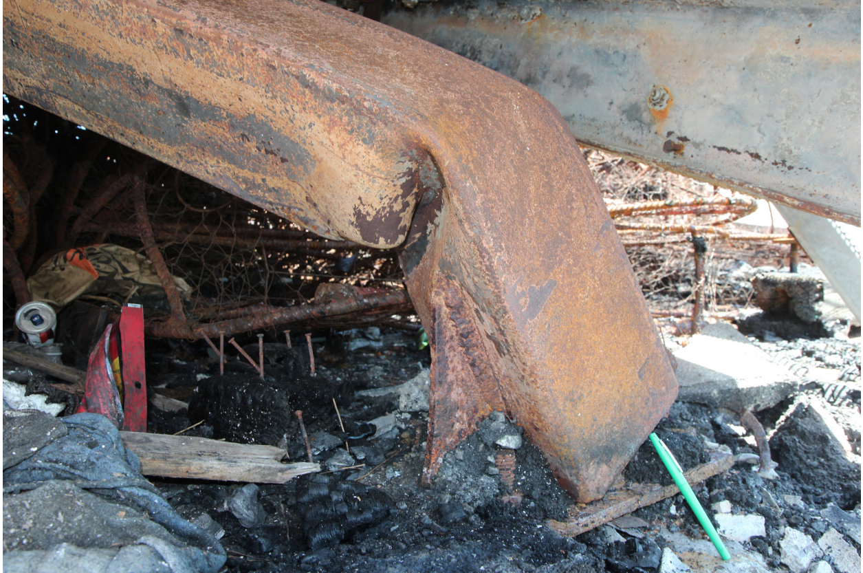
Figure A.30: Buckling at the base of the HSS column section on the western side of the structure, indicating that the base plate pullout strength exceeded the section's flexural strength.
