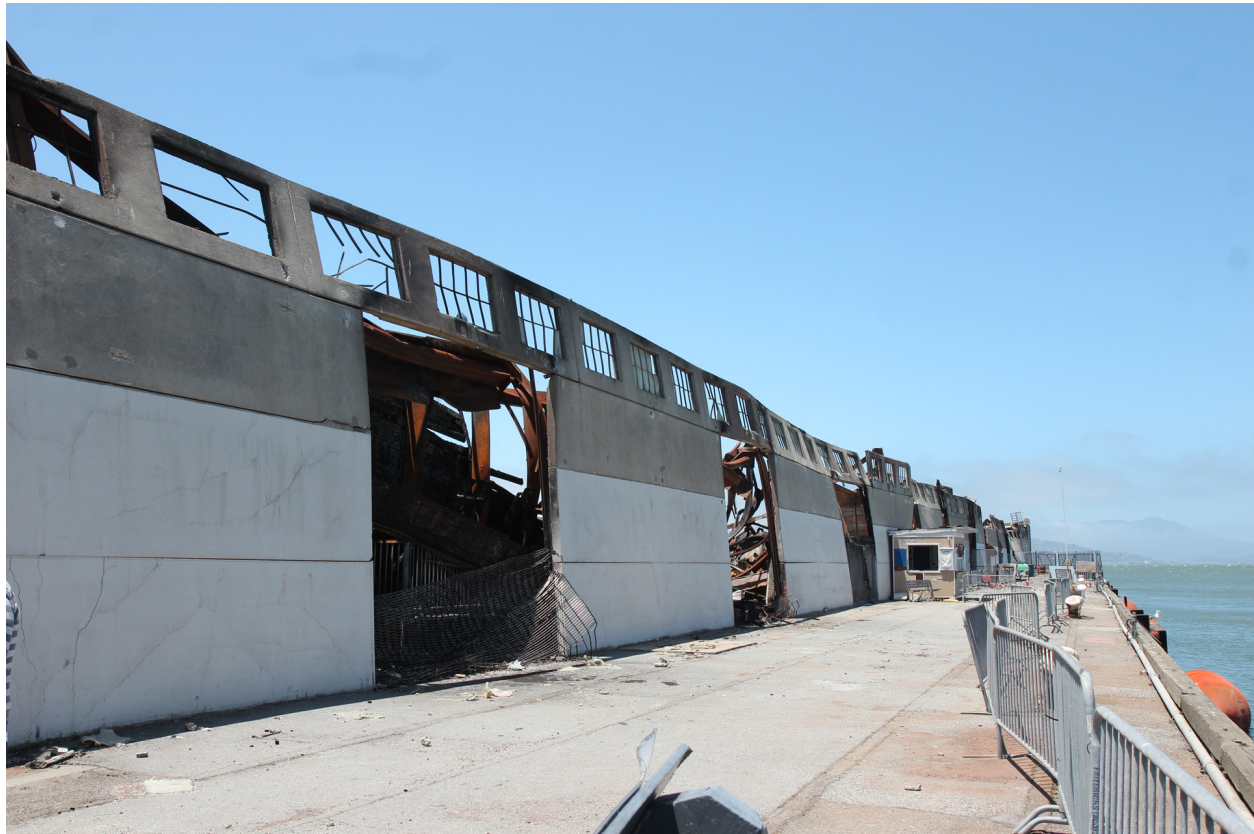
Figure 4.17: Damage to window and glass in east-side perimeter wall.
