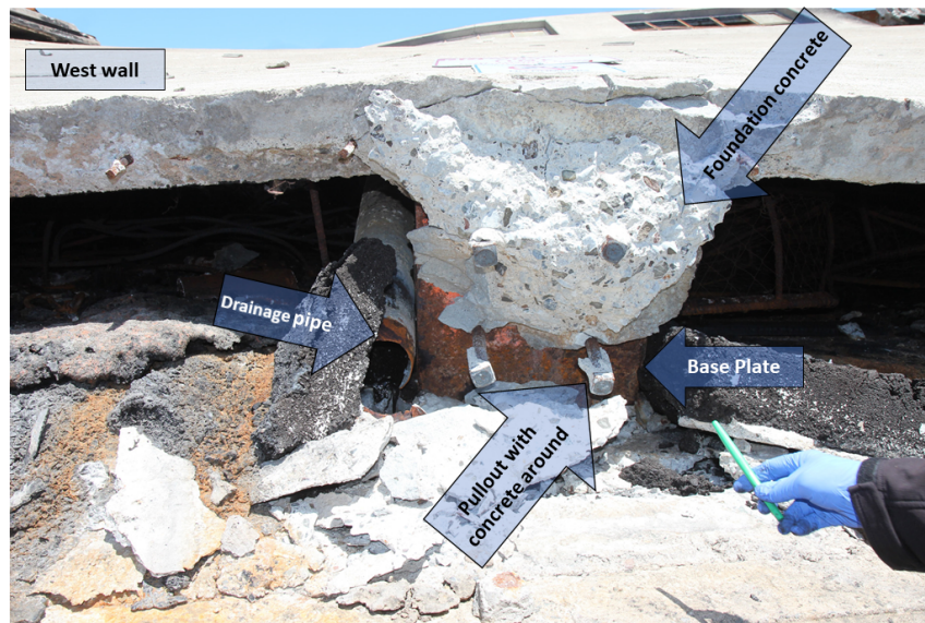
Figure 4.8: Failure of perimeter walls on the western part of the structure.
