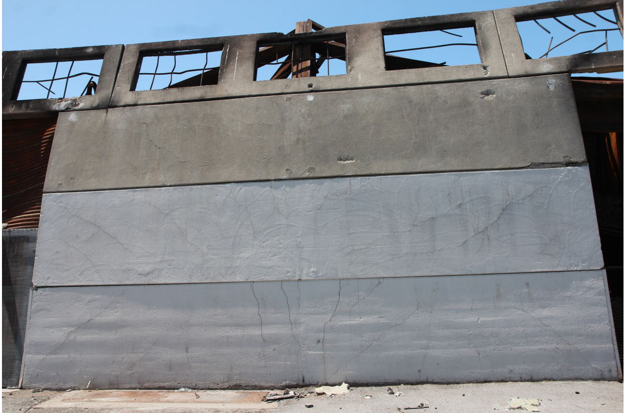
Figure A.27: Cracks in the concrete wall panel: diagonal at the edges and vertical at the center where the steel column provides support.
