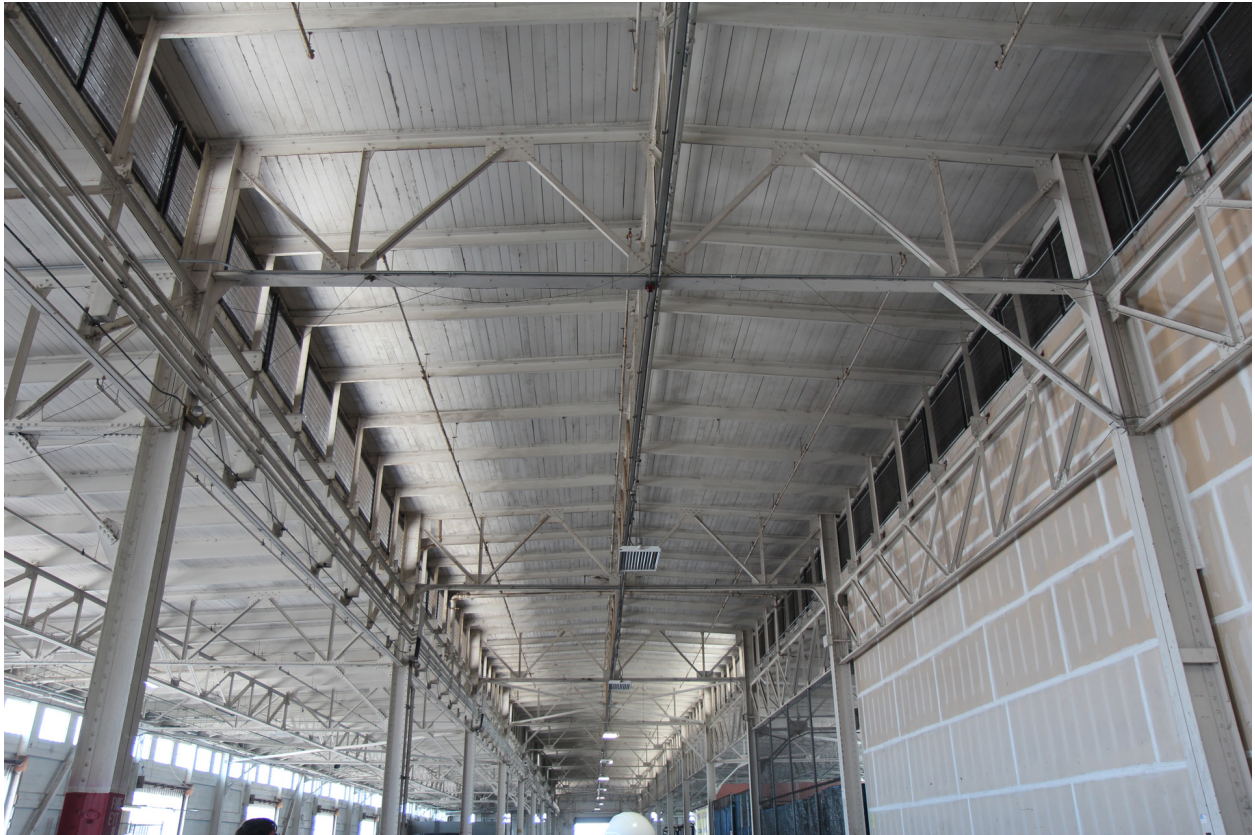
Figure 3.11: Undamaged condition of truss and roof of Shed A.
