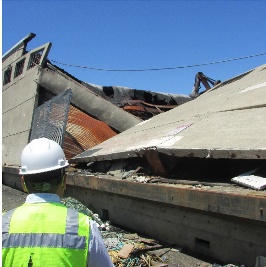
Figure 4.4: Overturning of the columns supporting perimeter walls on the western side of the structure.
