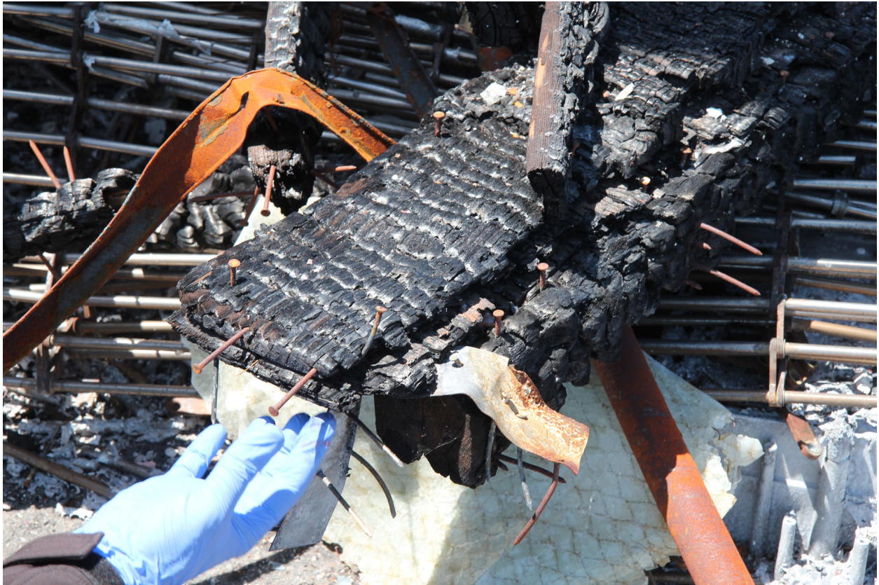
Figure 4.13: Timber roof charring from the east side of the structure.
