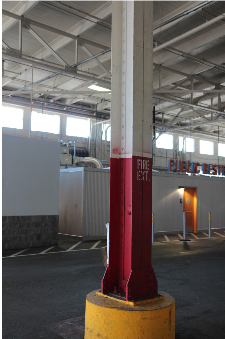
Figure A.1: A typical undamaged column in Shed A.
