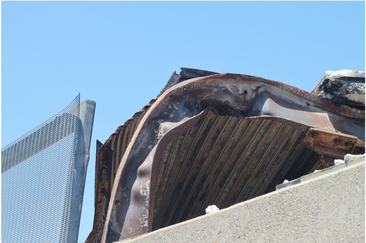
Figure A.21: Bending of column in the strong axis direction, with local buckling in the web.
