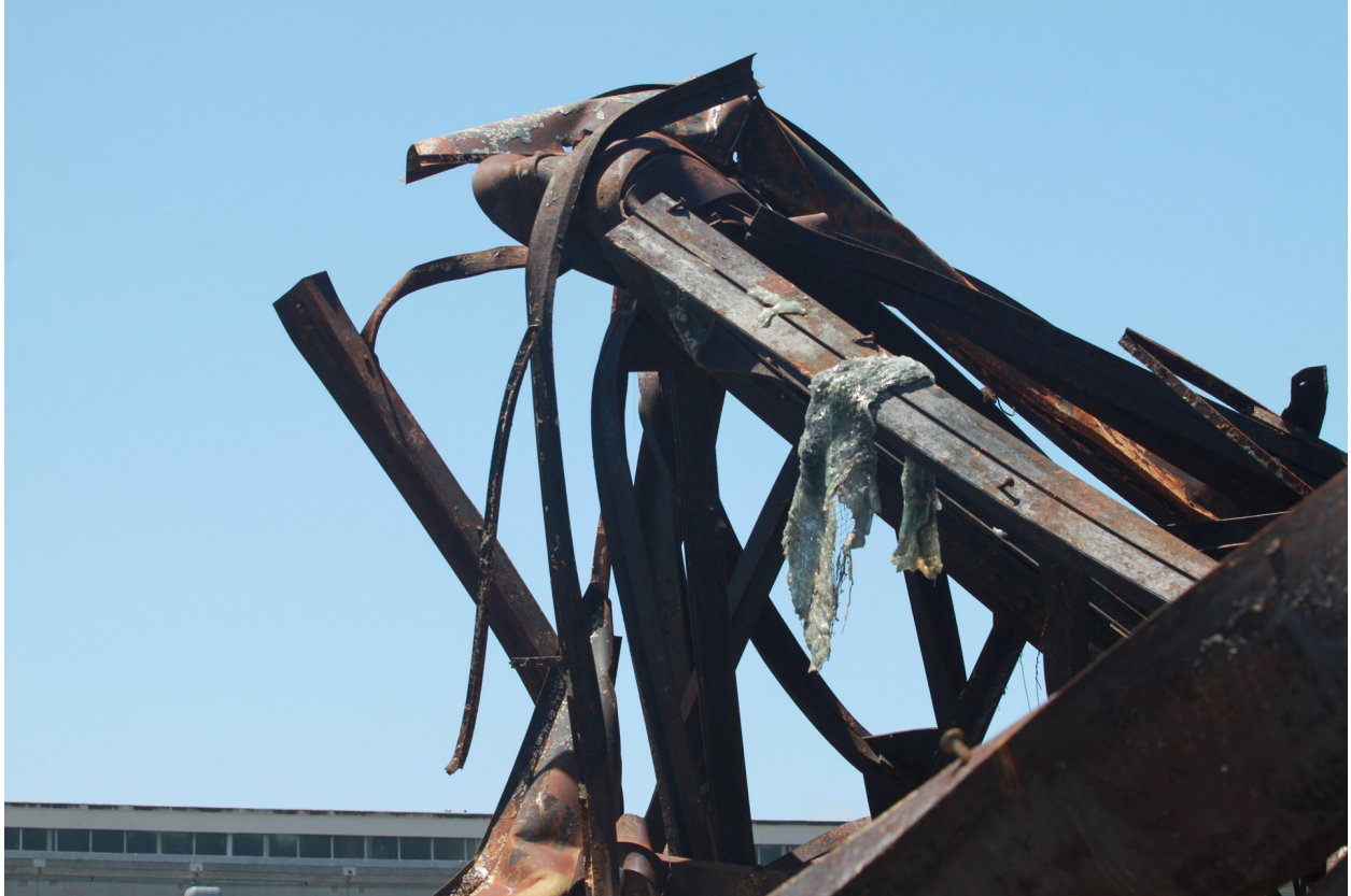
Figure A.29: Molten glass on steel members, about 10 ft from the east edge, indicating an inward collapse of the glass panels at some locations on the eastern side.
