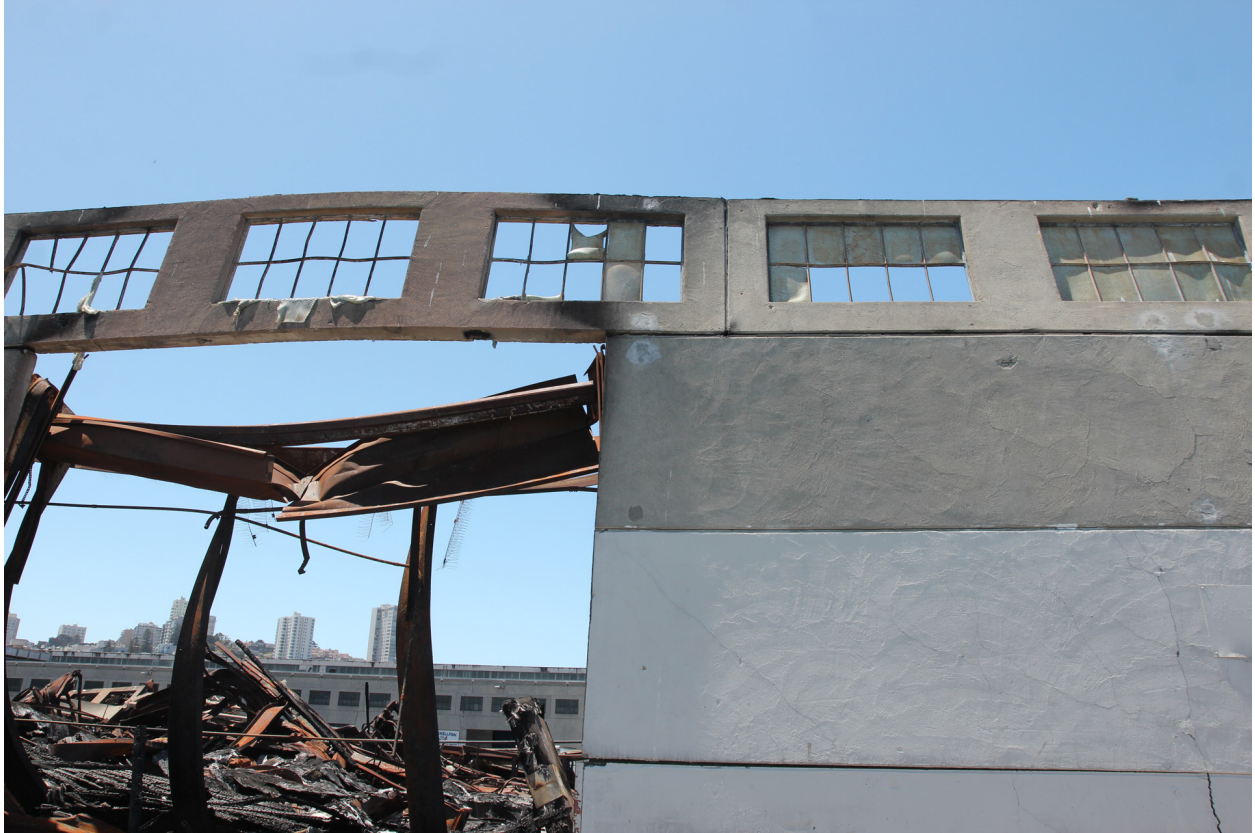
Figure 4.21: Severe glass damage on the top of opening (left) vs. limited damage on the top of concrete wall (right).
