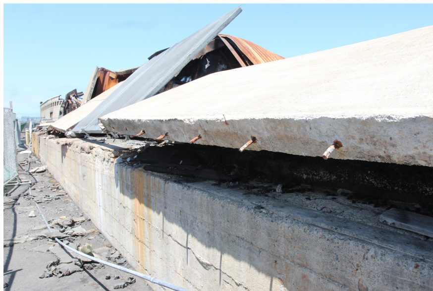
Figure 4.5: Failure of perimeter walls on the western side of the structure.
