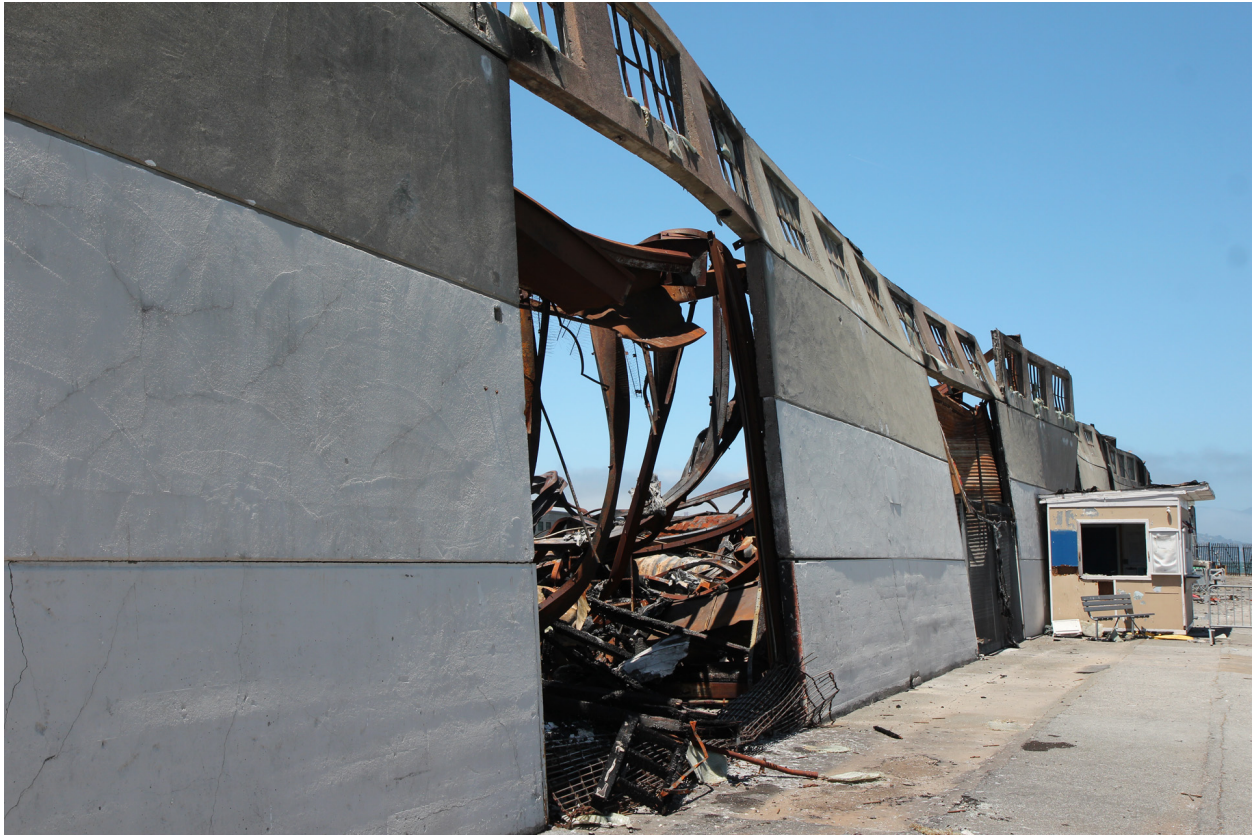
Figure 4.2: Damage on the east-side perimeter concrete walls and exterior columns.
