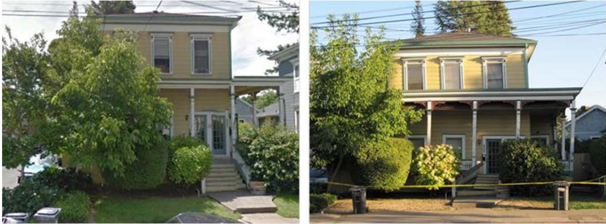
Figure 17 Before (left) and after (right) earthquake condition of the residential wood frame building with a cripple wall design in downtown Napa (Building H in the map in Figure 6).
