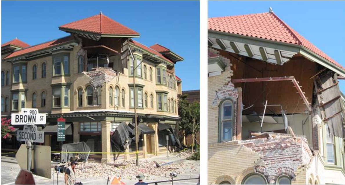
Figure 8 Overview of supporting column and walls at commercial building's top corner (Building B in the map in Figure 6).
