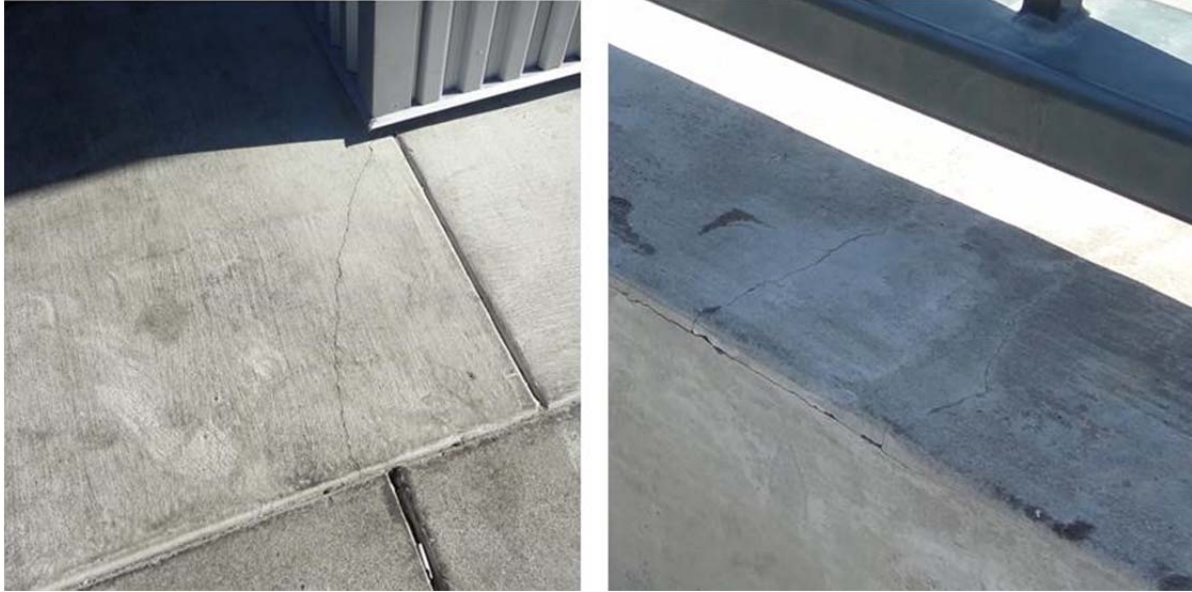
Figure 30 Cracking at various locations close to abutment of the First Street Bridge over Napa Creek from the Napa downtown side.
