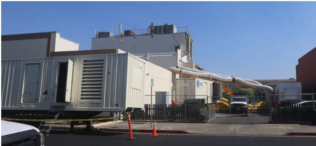
Figure 22 Failure of nonstructural wall at telecommunication center.
