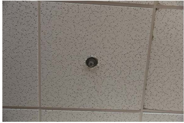
(b) Clearance for the fire sprinkler was exceeded
