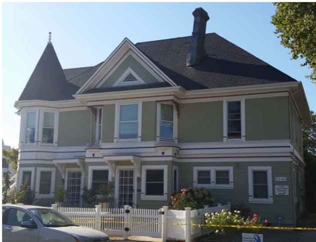
(a) Chimney leaning away from the street
