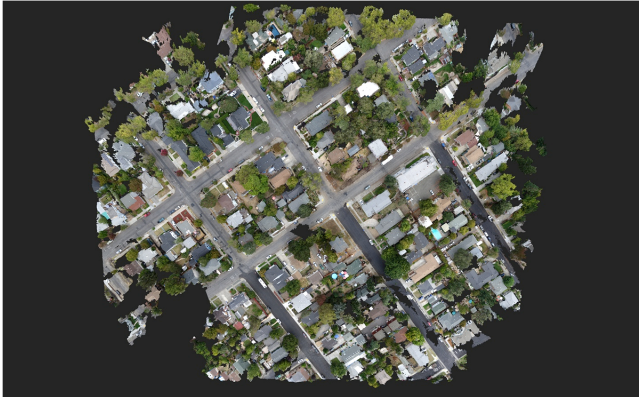
Figure 16 Reconstructed model of surveyed residential city block, capturing structural and non-structural damage to buildings and roadways.
