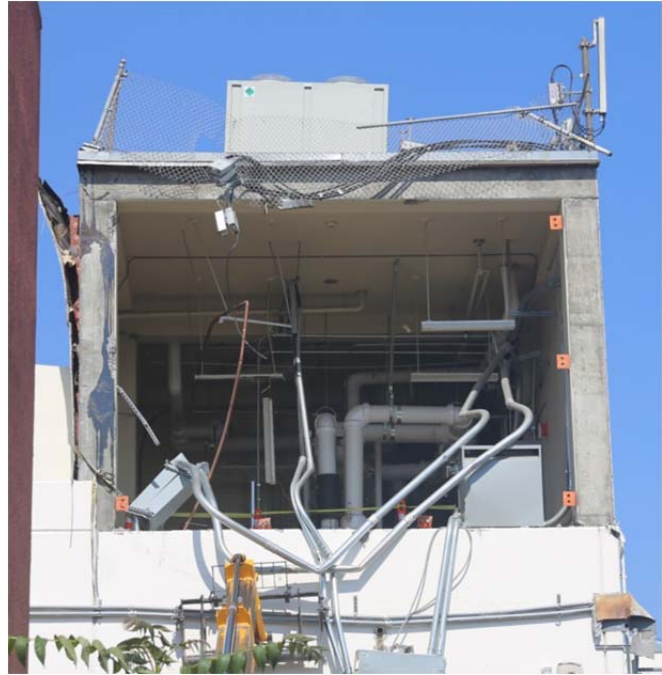
(b) Zoomed view of the brackets remaining in place; power conduits were damaged during the wall failure
