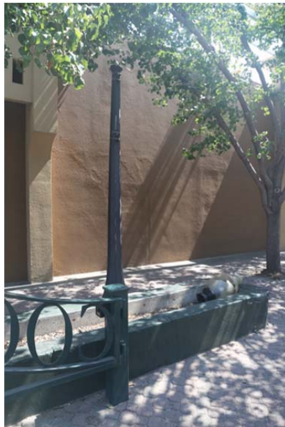
(a) Light fixture fell from the light pole
