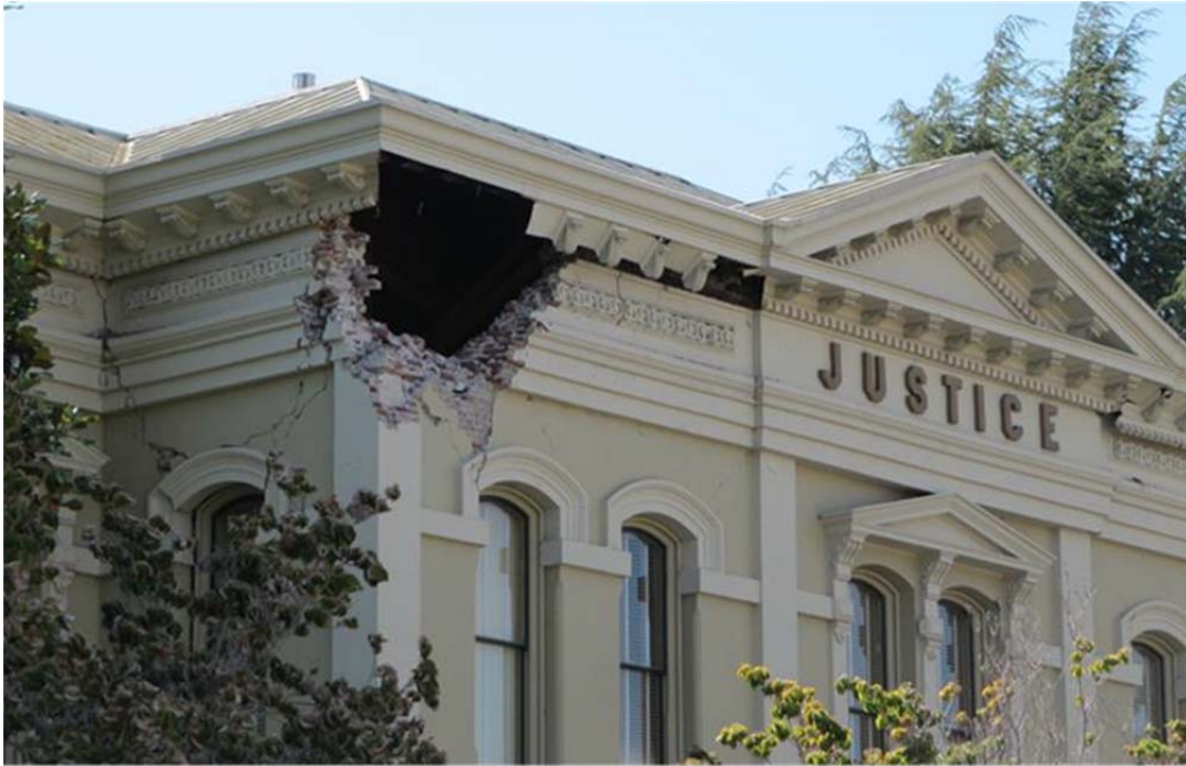
Figure 10 Damage and wide cracks in the top floor bearing wall of Napa Court House (Building D in the map in Figure 6).
