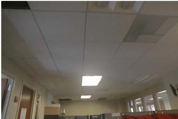
(a) Localized failures at the perimeter
