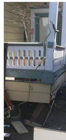
(b) Corner of the building
