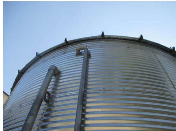
(b) Elbow of the pipe on right failed
