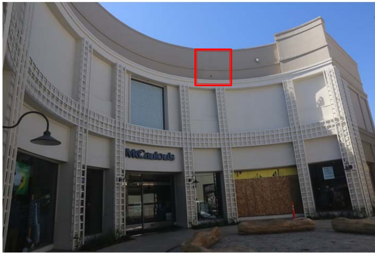
(a) Water pipe failed on the roof elevation and poured down through a hole in parapet (red square)
