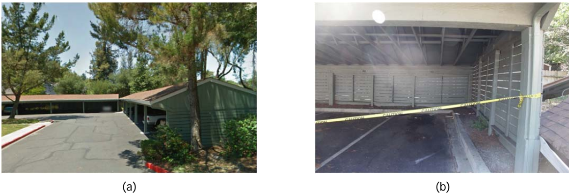
Figure 47 (a) Carports facing northwest before earthquake (Google Maps); and (b) Non-collapsed carport showing the roofing and wall system.
