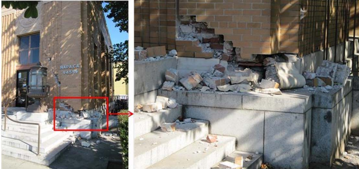
Figure 12 Damage in the south lower corner of Napa Post Office Building (Building E in the map in Figure 6).
