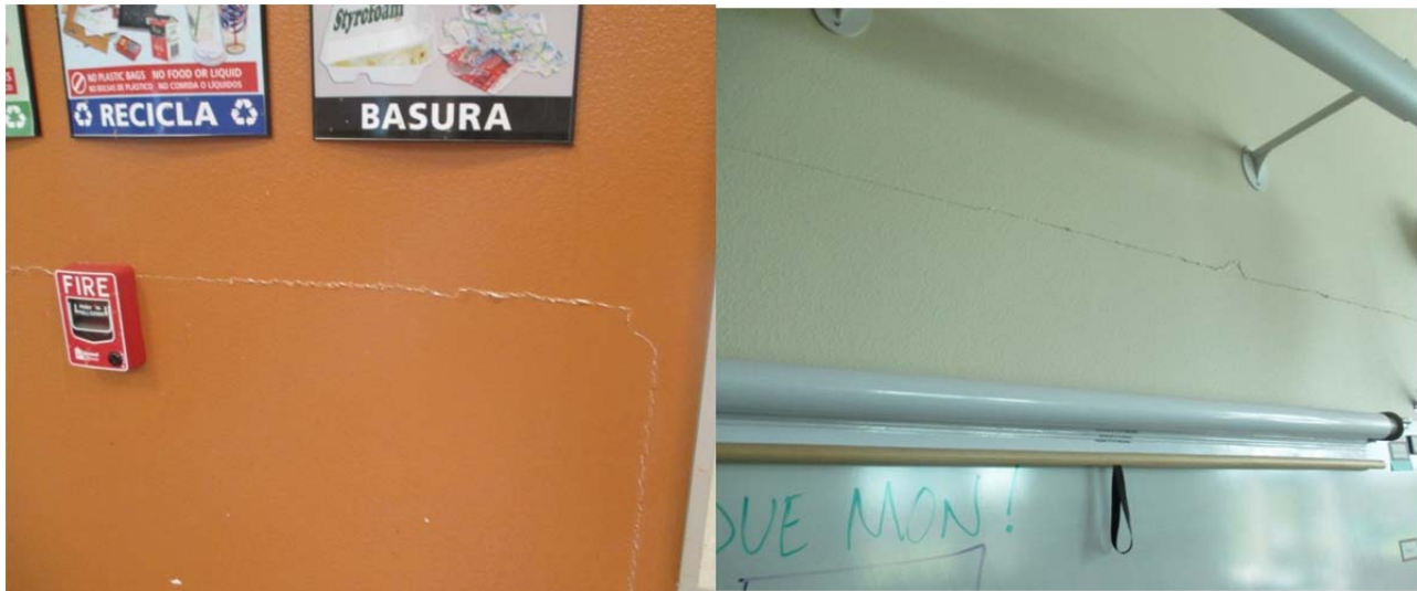
Figure 33 Wide spread tearing marks in gypsum board on walls mostly at horizontal joints.
