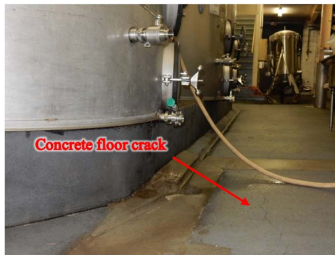
Figure 42 Cracking of concrete floor along the length of structure C, the 1989 addition for wine tank storage.
