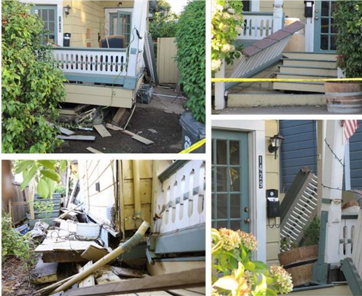
Figure 19 Close-up view of the cripple wall collapse at the east side of the building (top left) separation and elevation change in the main building's entrance stairs (top right) and patio fence (bottom right) utility ducts and pipes damage (bottom left).
