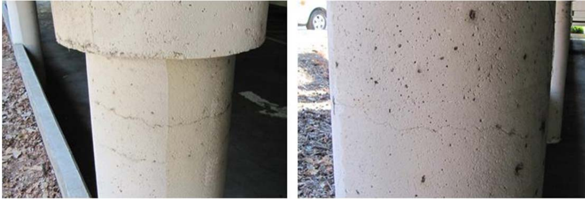
Figure 20 Flexural cracks in basement floor columns of multi-story RC garage building (Building I in the map in Figure 6).
