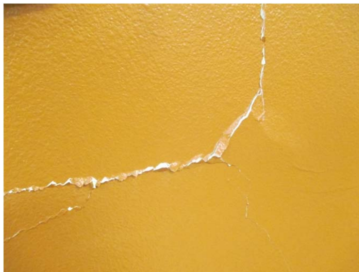
Figure 32 Tear in gypsum board on walls.
