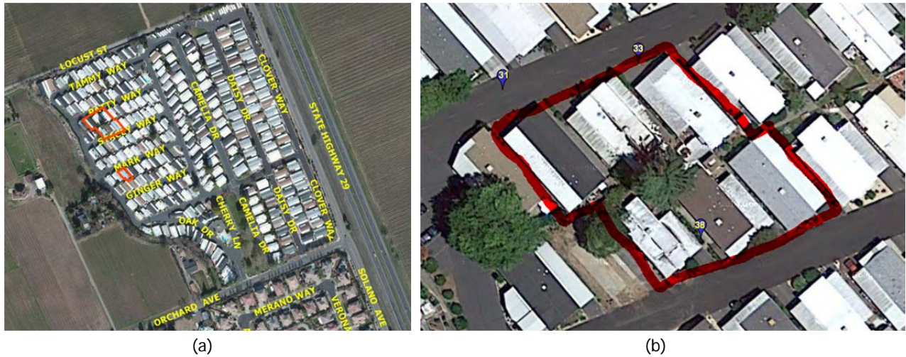
Figure 2 (a) NVMHP Park and locations of fires, 24 Aug 2014 S. Napa M_w 6.0 earthquake; and (b) 317 Patty Way fireground, showing locations of photos 31, 33, 38 in Figs. 3 and 4 (damaged buildings outlined in red).
