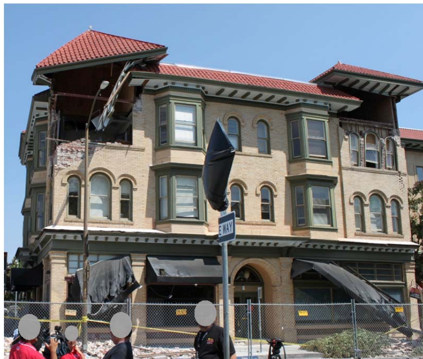
Figure 9 Partial collapse at 1001 2 nd Street.
