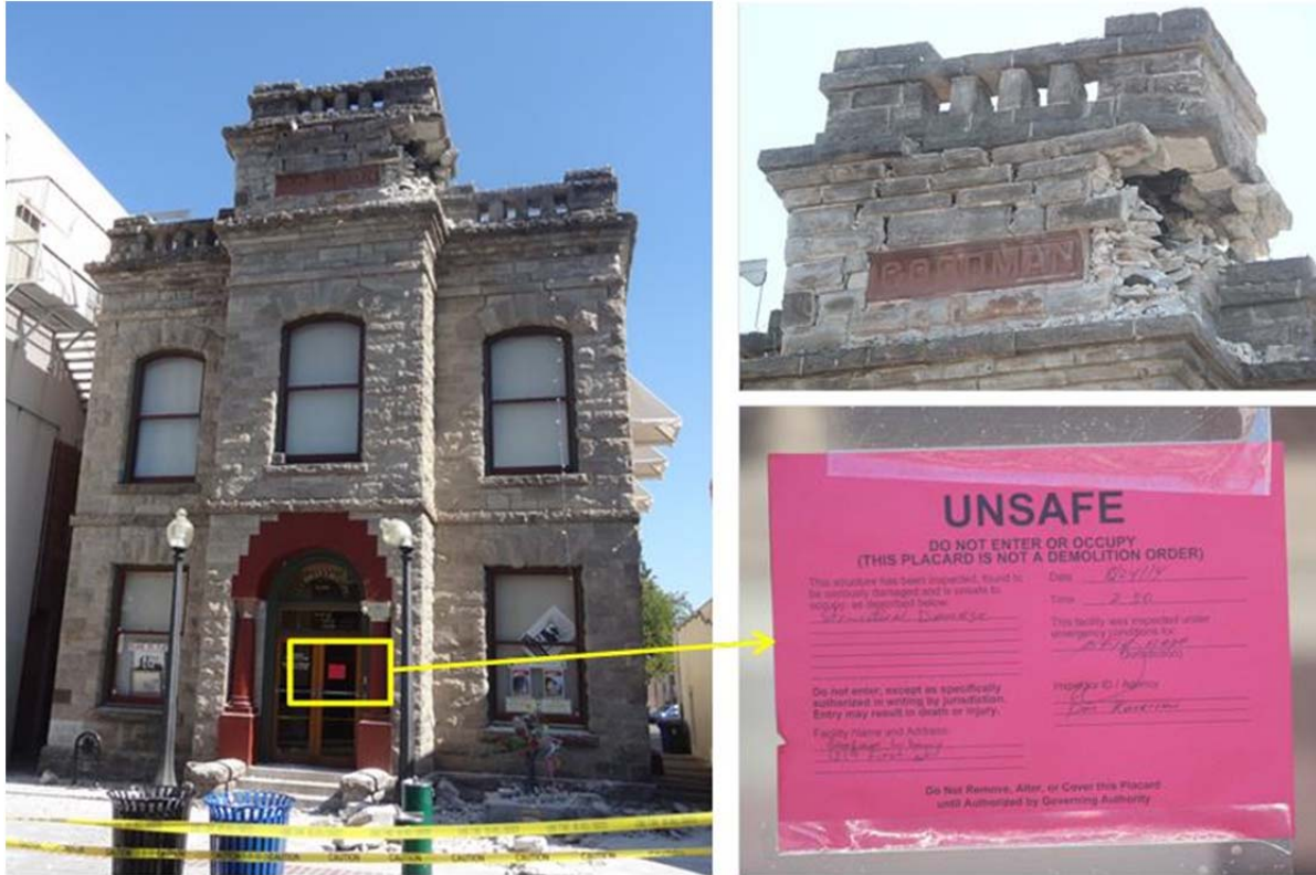
Figure 7 Overview of Goodman historical library building (Building A in the map in Figure 6) and red tag displayed at the building's entrance.
