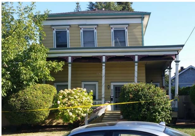
(a) Global view after the earthquake
