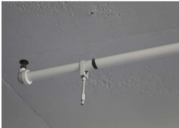
(a) Failure of the ceiling anchor
