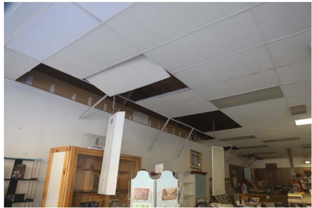
(b) Failure concentrated around perimeter on floating side
