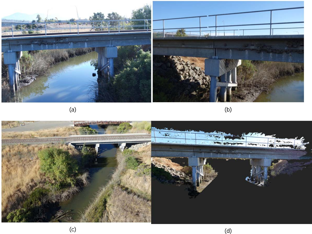
Figure 23 (a) Ground view; (b) aerial close up view; (c) aerial view of bridge; and (d) reconstructed model.
