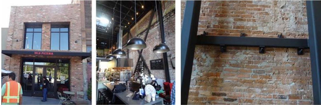
Figure 22 Example of a retrofitted UMB using a steel braced-frame that performed well during the earthquake with no signs of any structural or nonstructural damage.
