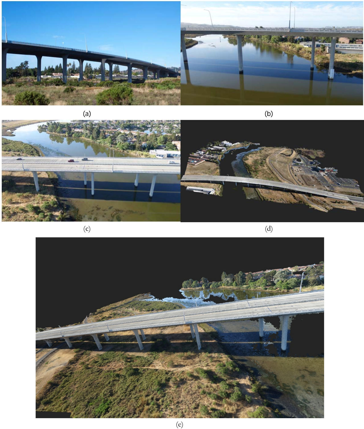
Figure 20 (a) Ground view; (b) aerial view from low altitude; (c) aerial view from high altitude; (d) complete reconstructed model of bridge; and (e) close up of reconstructed model.
