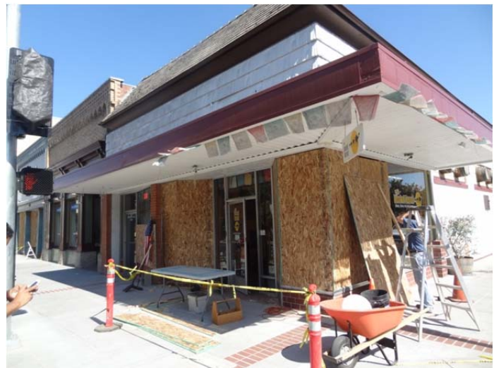
(b) The majority of glass windows of the first floor failed
