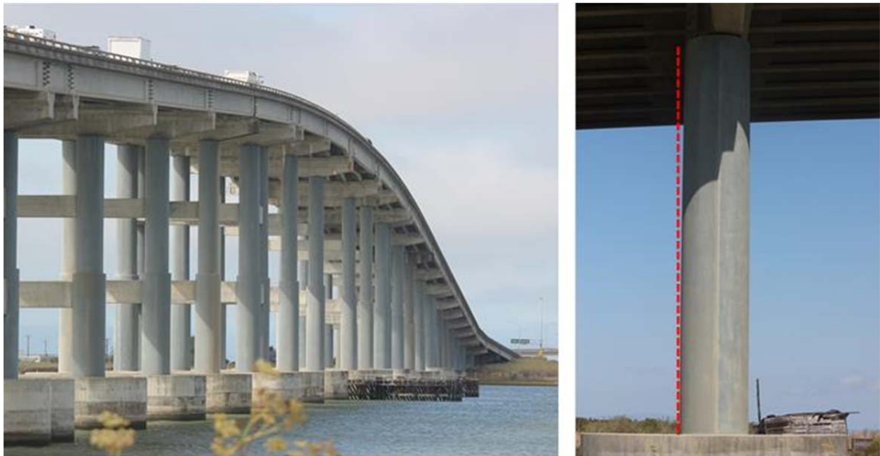
Figure 27 Overview of CA-37 Vallejo bridge (left) and suspected pier tilt close to the bridge approach from the Mare Island side (right).
