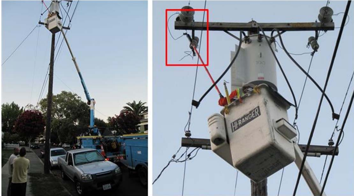
Figure 25 Efforts to fix wires and connections failures in local street power distribution lines.
