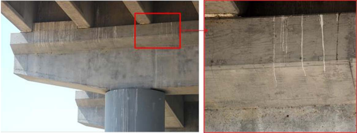
Figure 28 Cracking of one of the bridge piers' cap beam flange.
