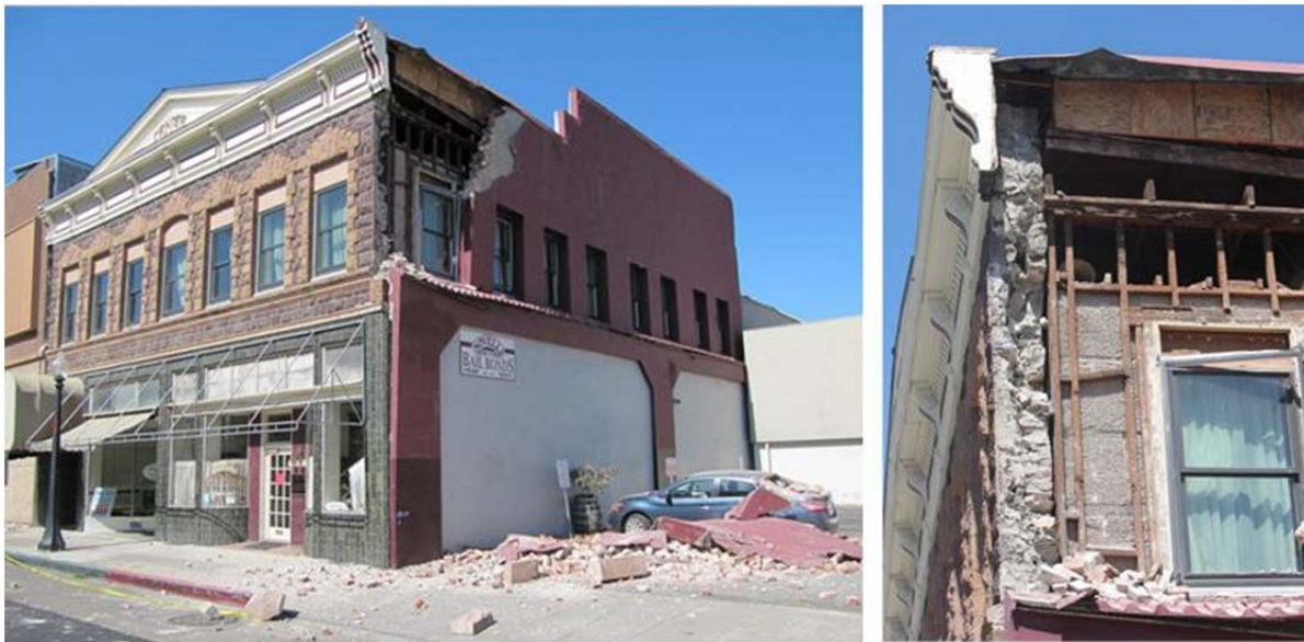
Figure 9 Overview of side wall collapse of a commercial building leading to a the damage of a car parked next to the building (Building C in the map in Figure 6).
