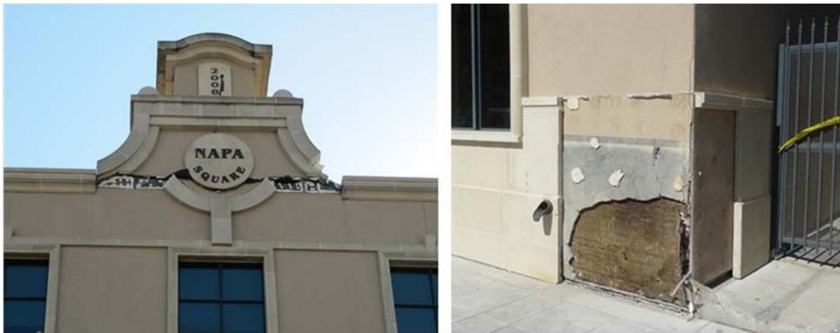
Figure 24 Damage in shopping mall façade in downtown Napa.
