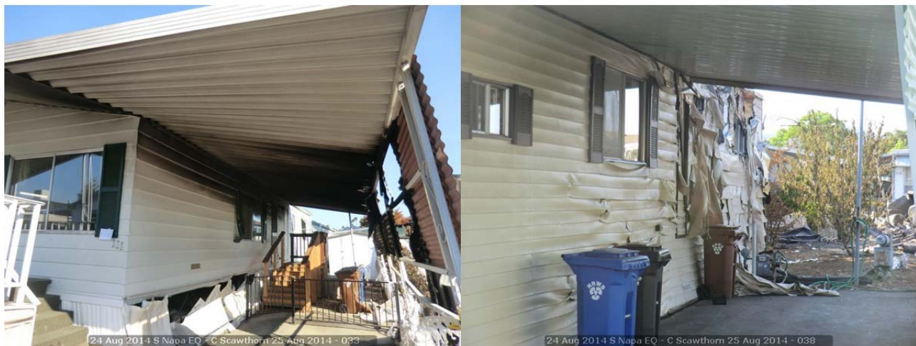
Figure 4 Damage to exposure structures, 317 Patty Way, NVMHP Park, 24 Aug 2014 S. Napa M_w 6.0 earthquake: (a) structure to east of fireground; and (b) structure to south of fireground.
