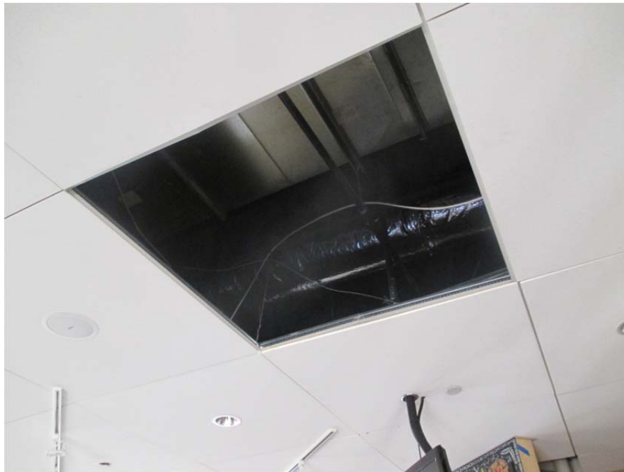
Figure 13 Large 4 ft by 4 ft ceiling panel failed during the earthquake.
