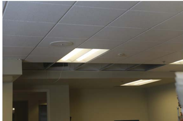
(b) Localized failures at the perimeter
