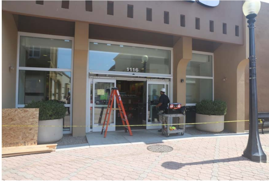
Figure 29 Damaged door is under urgent repair.
