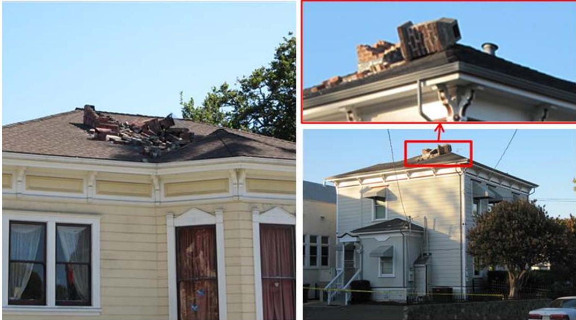
Figure 23 Damage of residential buildings chimneys in downtown Napa (Buildings shown are Building J (left) and K (right) identified in map in Figure 6).
