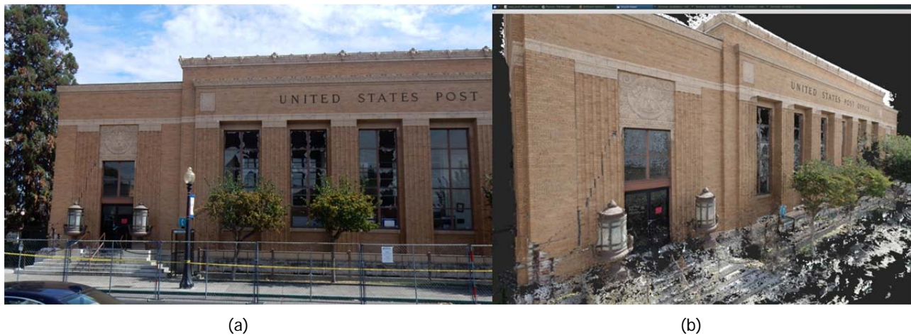
Figure 8 (a) Ground view of post office; and (b) reconstructed model capturing façade and window damage.
