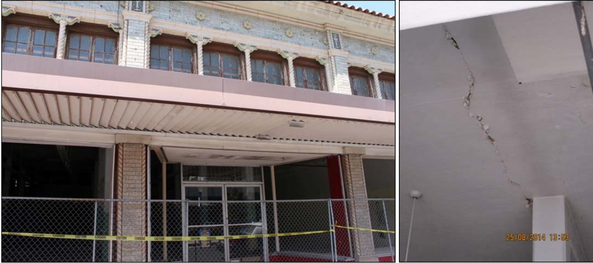
Figure 4 URM building at 1212 1 st Street.
