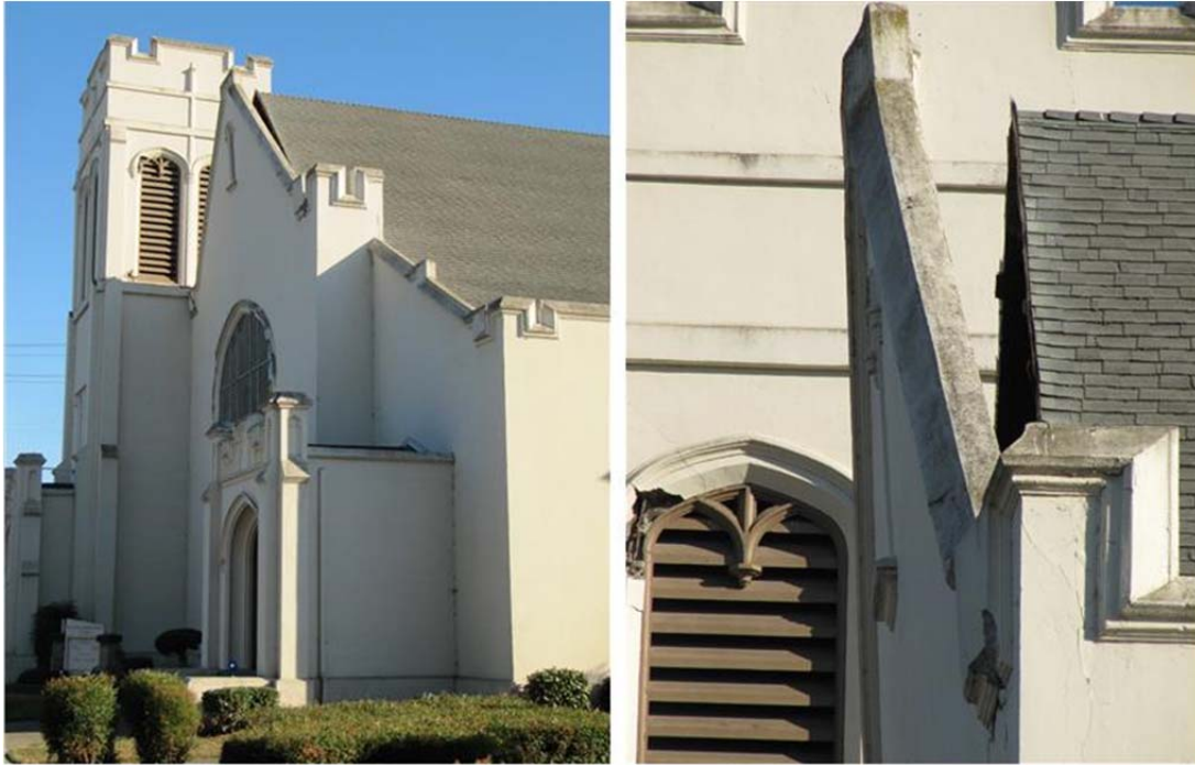
Figure 14 Separation gap between the church (Building F in the map in Figure 6) roof and the east wall in a global (left) and zoomed-in (right) views.
