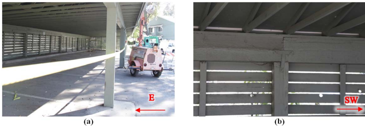
Figure 50 Details for Carport #7: (a) view looking southwest along longitudinal wall; and, (b) yielded connection of a rear-interior column and roof system showing permanent displacement to the southwest.
