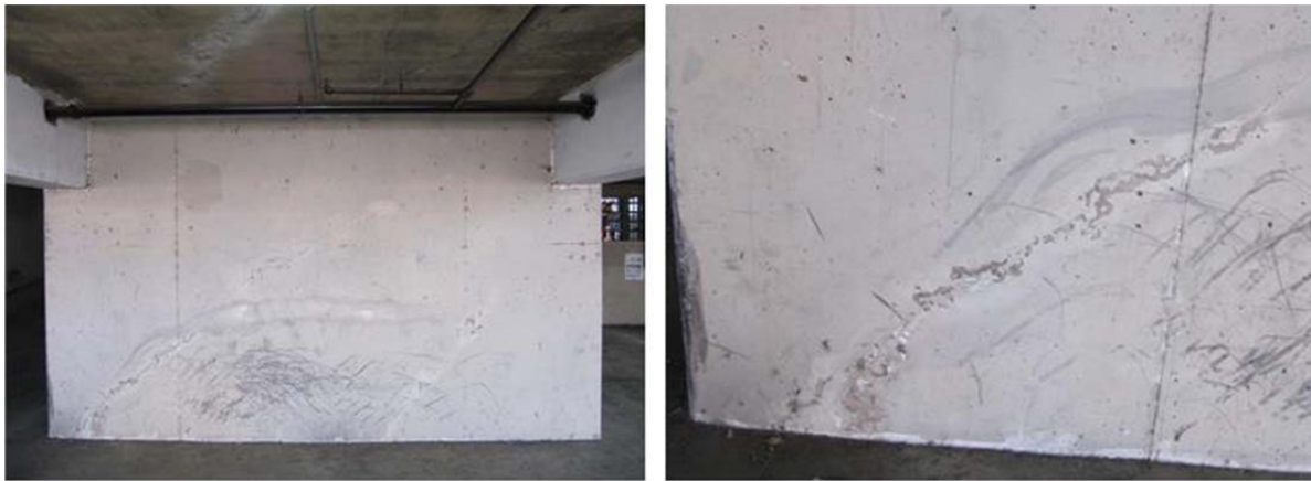
Figure 21 Minor diagonal cracks in basement floor shear wall of multi-story RC garage building (Building I in the map in Figure 6).
