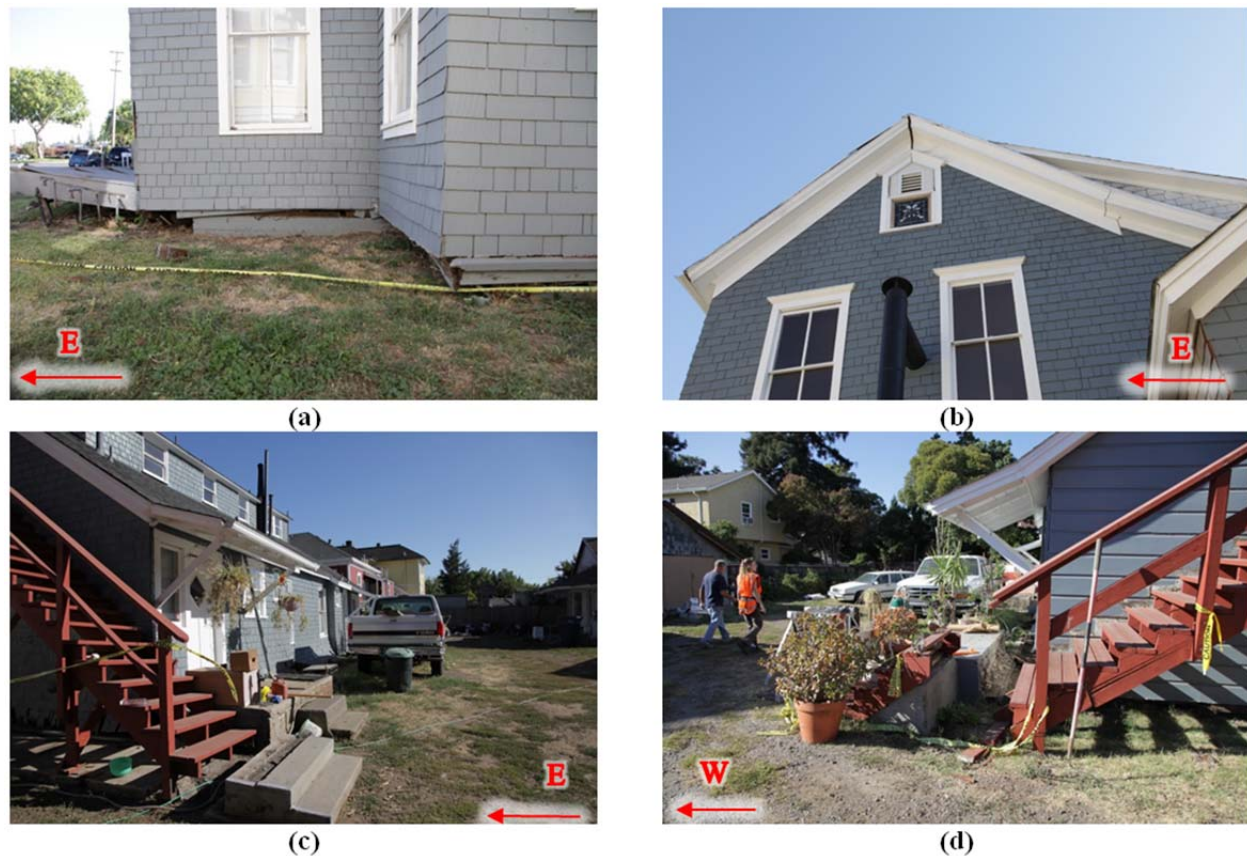
Figure 54 Details of damage at red-tagged residence at 1251 Jefferson Street: (a) collapsed cripple wall and relative displacement between foundation and super-structure of approximately 0.3-0.6 m; (b) crack at roof ridge due to translation of superstructure off of the foundation; (c) displacement of wooden staircase and concrete foundation stairs; and (d) vertical and horizontal displacement of superstructure observed at the rear doorway and staircase.
