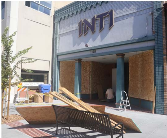
(a) All glass windows failed in a small business
