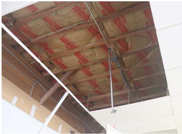
(a) No brace wires were installed
