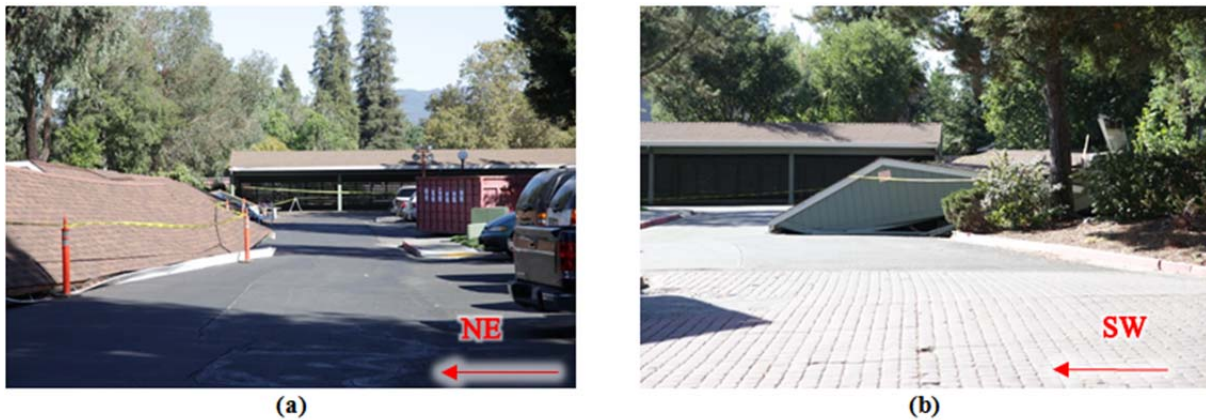
Figure 48 Views of carports post-earthquake showing collapsed and non-collapsed carports facing; (a) Southeast and (b) Northwest.
