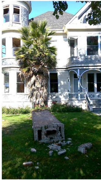
(a) Massive chimney that fell away from the house to the ground
