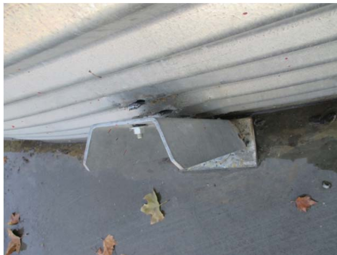
Figure 30 Base anchorage separated from the tank wall.
