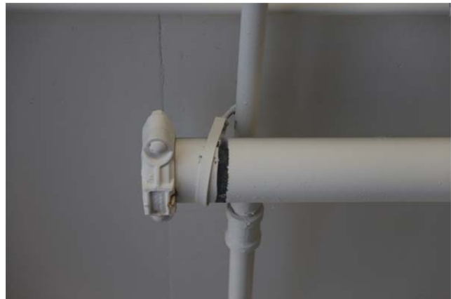
(b) Residual deflection of a pipe
