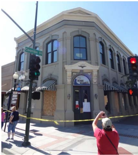
(c) Glass broken on both sides of the two-story building (torsional effect)
