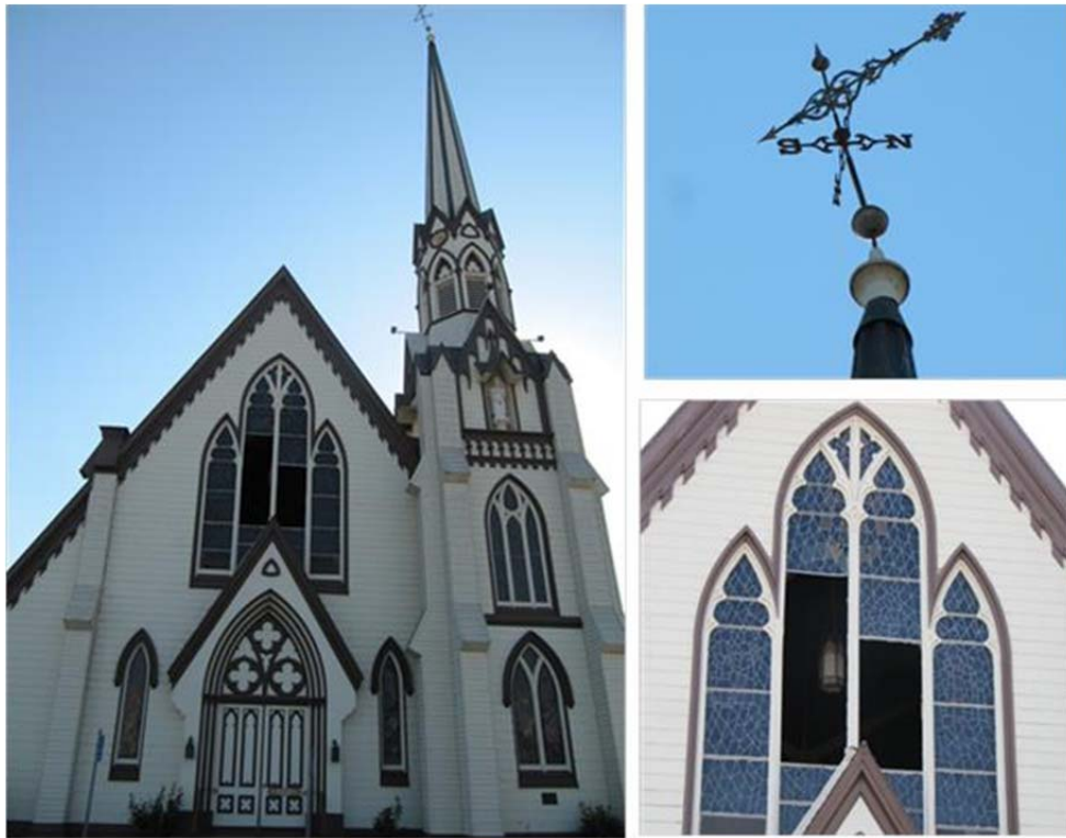
Figure 15 Overview of historic church (Building G in the map in Figure 6) non-structural damage: façade smashed windows and deformed top cross.
