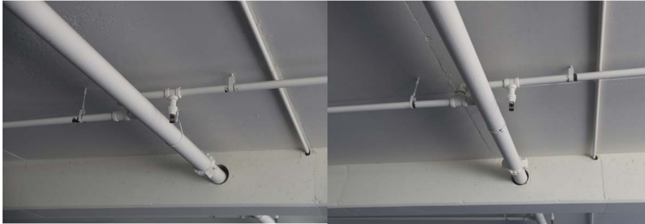
(a) Scratches on the pipes show the amplitude of motion within a supporting bracket (larger for a largely oversized access hole)
