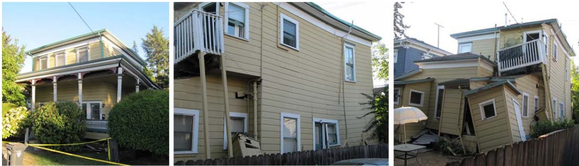
Figure 18 Global views of different sides of an old residential wood building (Building H in the map in Figure 6).
