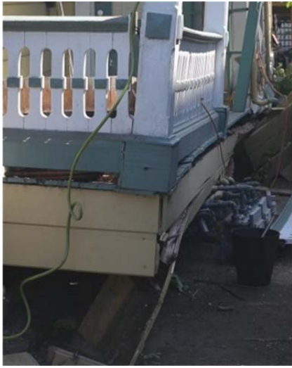
(a) Photo of collapsed porch
