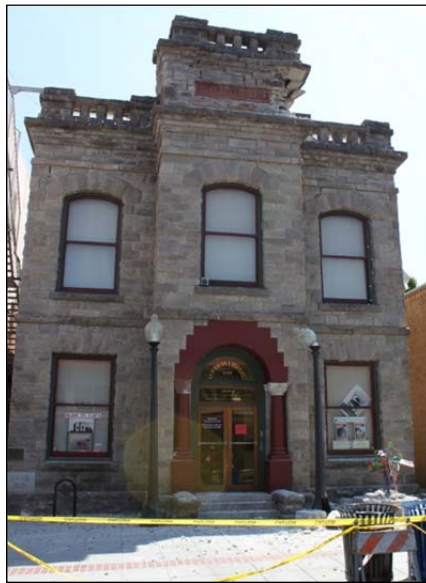
Figure 3 URM building at 1219 1 st Street.
