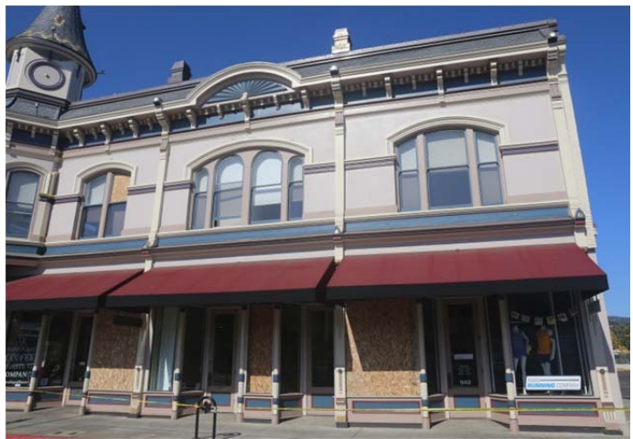
(b) The majority of glass windows of the first floor failed
