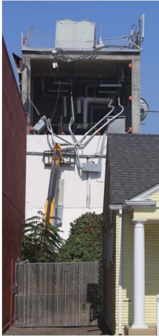
(a) Nonstructural wall suspended on brackets (orange) failed
