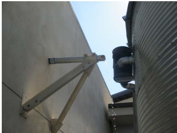
(a) Rain leader pipe roof failed
