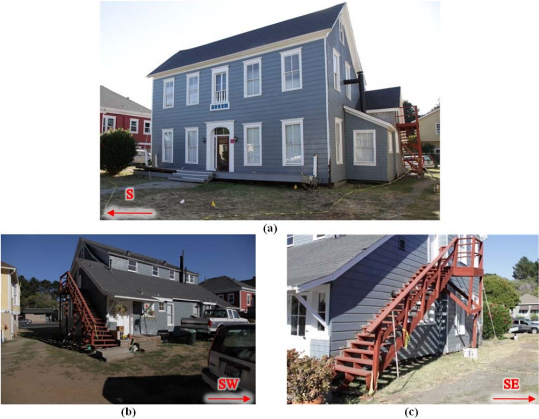
Figure 53 Red-tagged residence at 1251 Jefferson Street: (a) view from Jefferson St; (b) view of dislocated stairs from backyard facing east-southeast; and (c) view of stair damage from backyard facing east-northeast.
