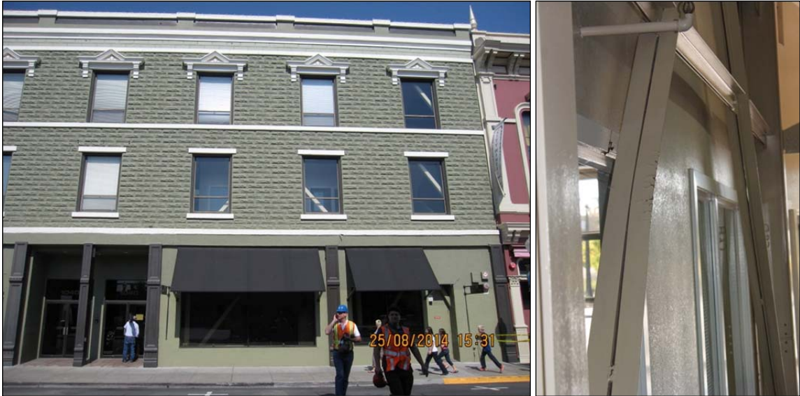
Figure 6 URM building at 1040 Main Street.
