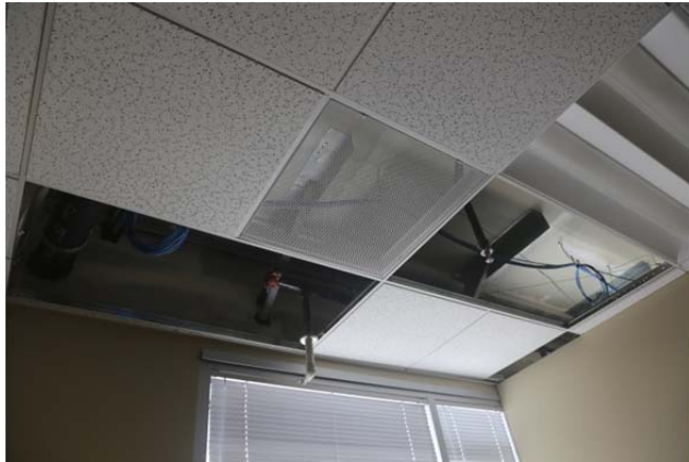
(a) Failure of a panel due to interaction with fire sprinkler
