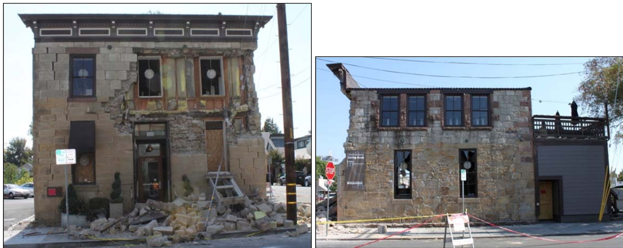
Figure 1 URM building at 1245 Main Street.
