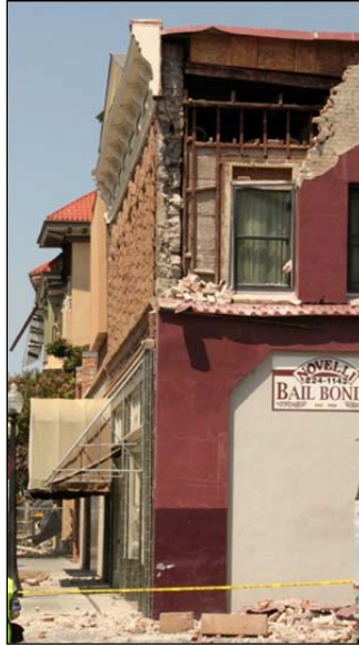
Figure 2 URM building at 810 Brown Street.
