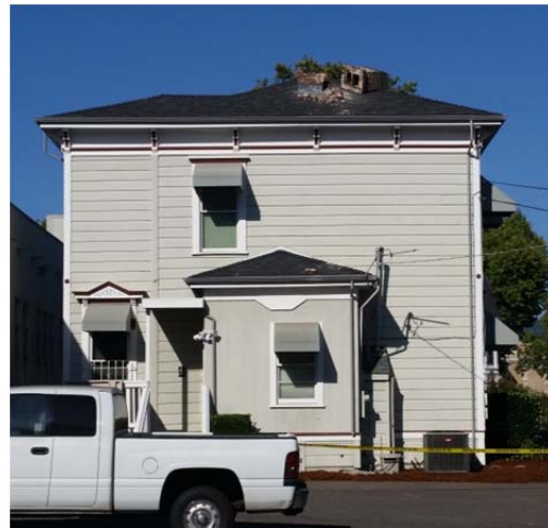
(b) Complete failure with pieces still on the roof
