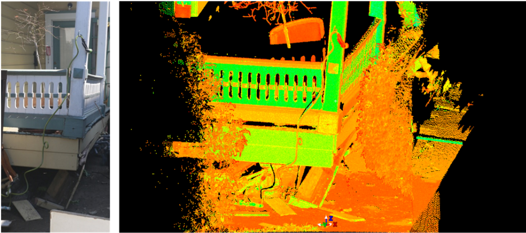
Figure 35 After condition of the wood frame building with a cripple wall design.
