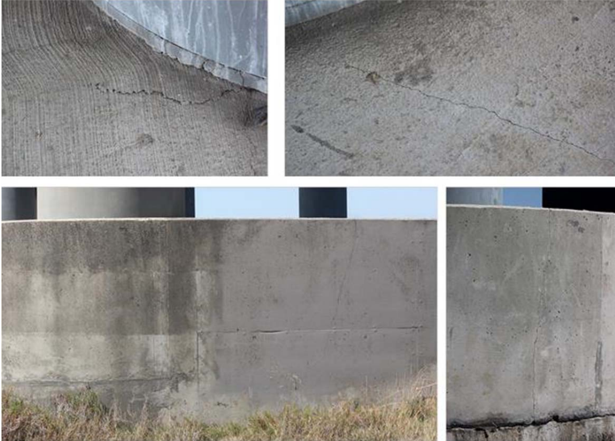
Figure 29 Cracking of one of the bridge pier's pile cap.
