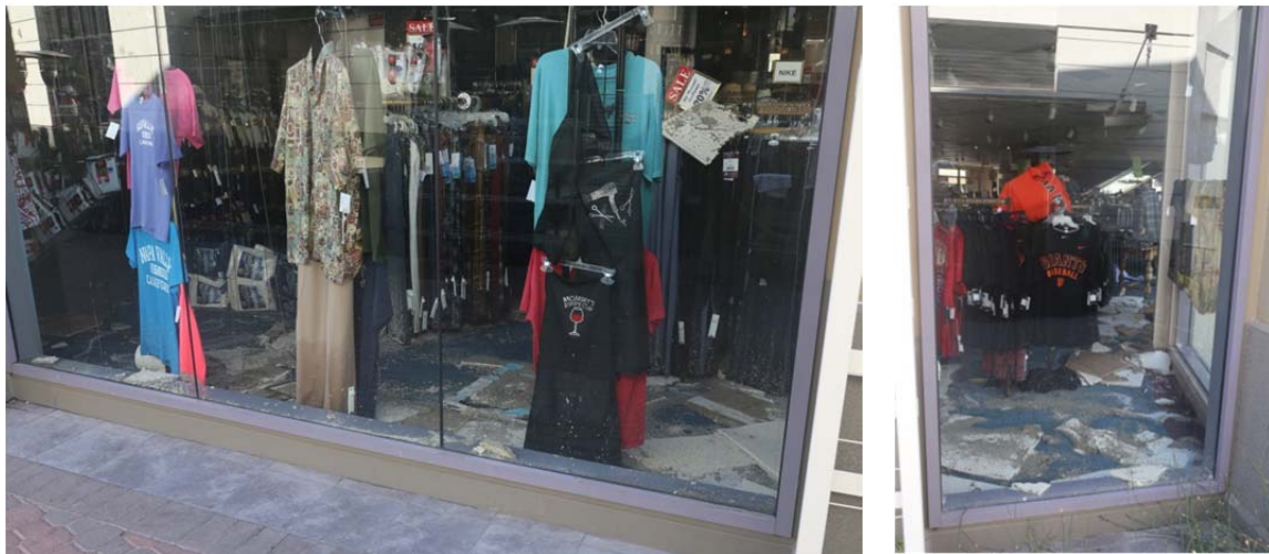
Figure 18 Soaked suspended ceiling tiles and goods on the floor.
