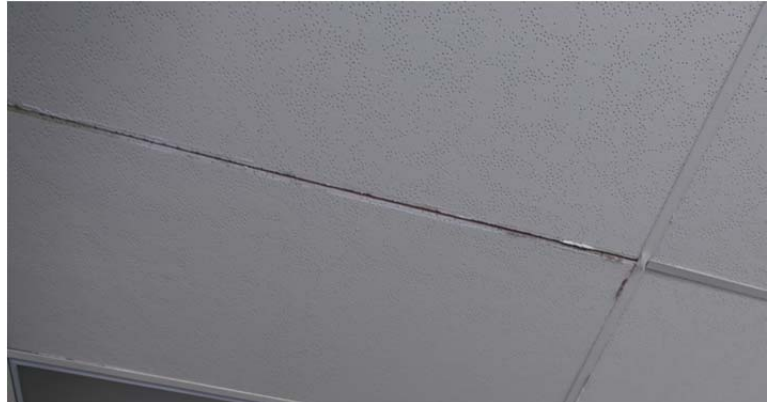
(b) Missing tee-bar failure
