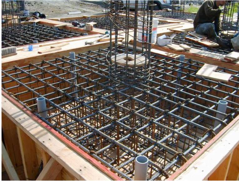
**Fig. A.16 Anchor block reinforcement cage.**
