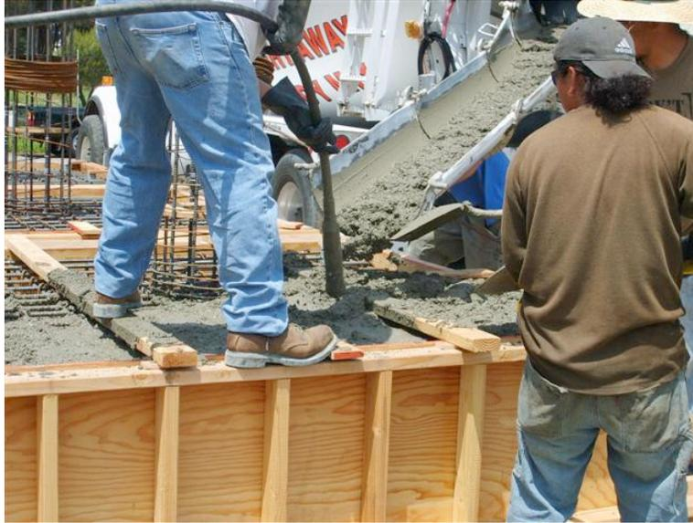
**Fig. A.17 Casting anchor block.**
