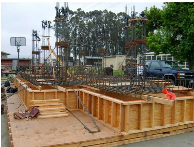
**Fig. A.15 Placement of longitudinal bars.**
