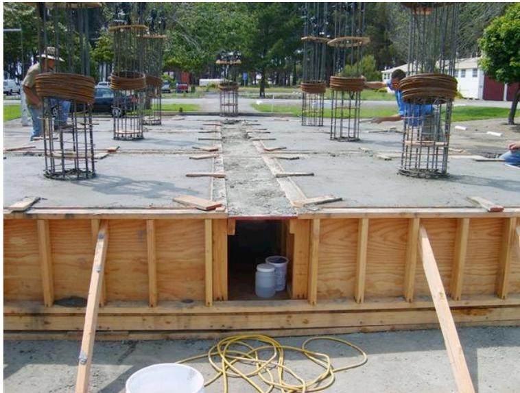
**Fig. A.18 After casting the anchor blocks.**
