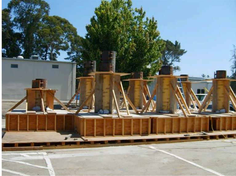
**Fig. A.21 Installation of steel jackets.**
