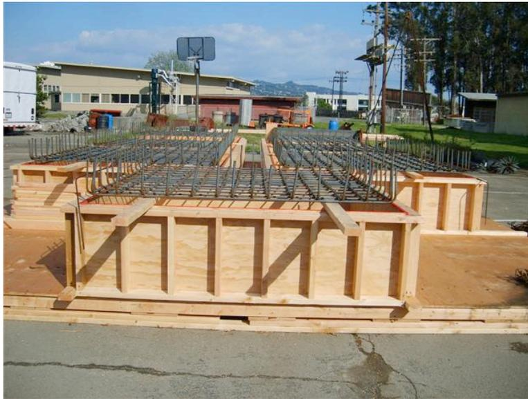
**Fig. A.14 Bottom portion of anchor block cage.**
