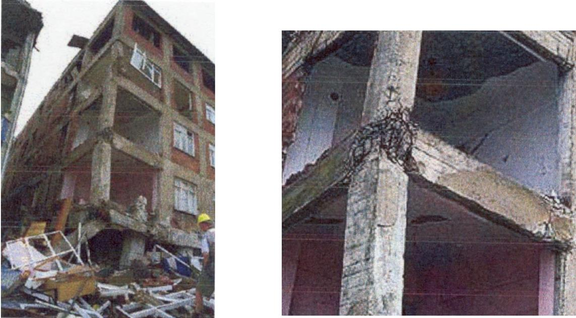
**Fig. 1.1 Collapse of a building by joint shear failure (Sezen et al. 2000).**
