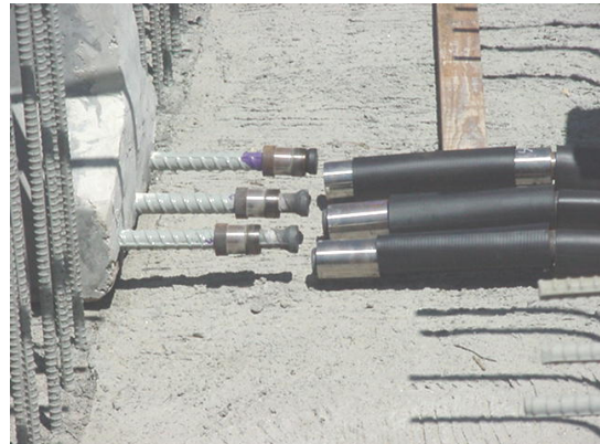
Fig. 15. Mechanical couplers for main girder reinforcement.
