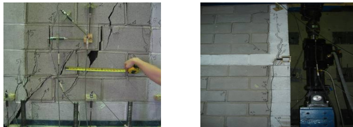
Fig. 5. Cracking and failure mode of partially grouted walls [9].
