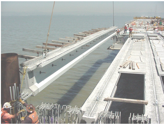
Fig. 11. Pre-cast girders placed in cap beam openings.
