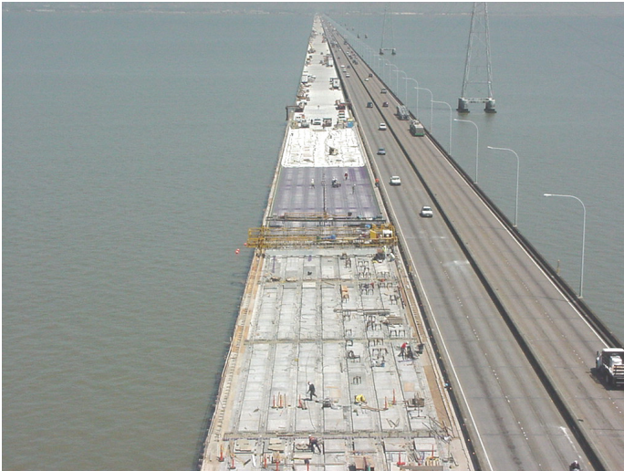
Fig. 17. San Mateo bridge near completion.
