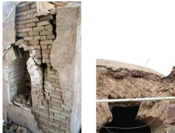
Fig. 7. Effective reaction of arched openings.
