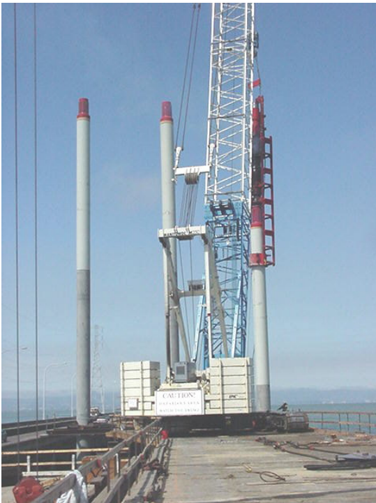
Fig. 7. 42-inch hollow shell column/shaft driving operation.
