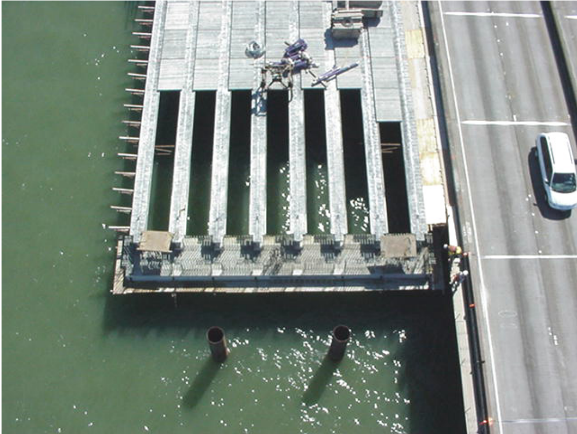
Fig. 13. Top view of pre-cast bridge components.
