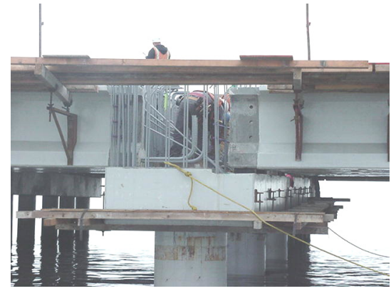
Fig. 12. All pre-cast elements placed in designated openings.
