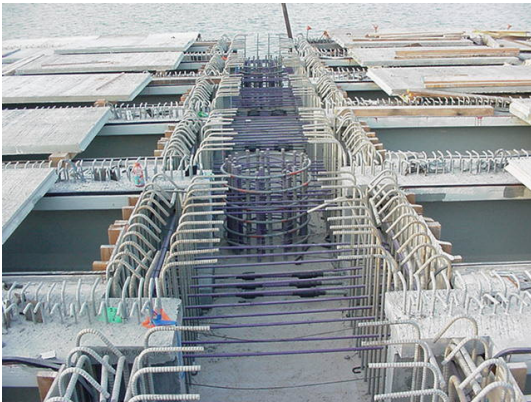
Fig. 14. Cast-in-place portion of bent cap beam ready for concrete pour.
