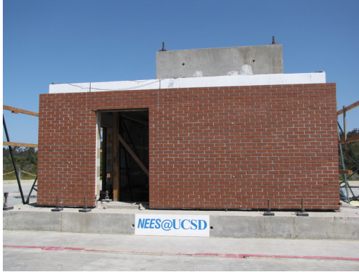
Fig. 3. Reinforced concrete masonry building, essentially undamaged after four incredible earthquakes.
