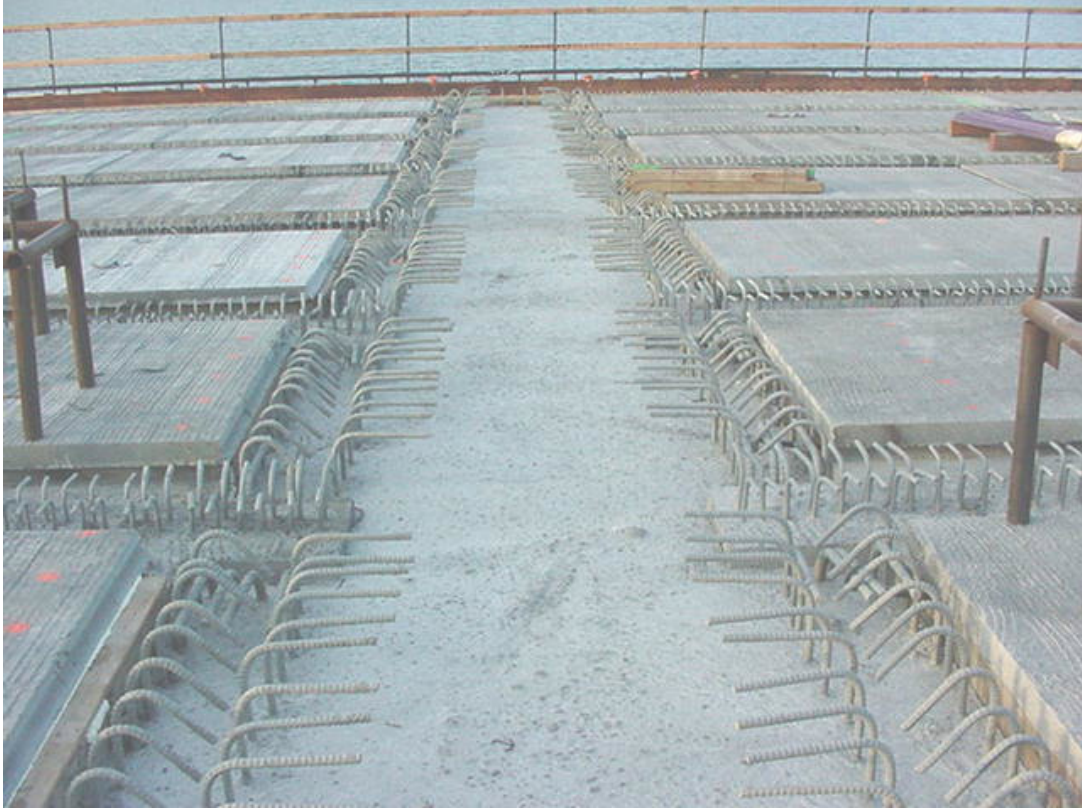
Fig. 16. View of completed bent cap beam ready for top reinforcement.
