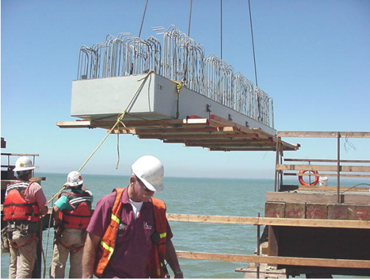
Fig. 9. Pre-cast portion of the bent cap beam.
