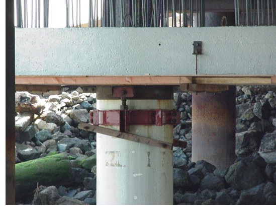
Fig. 10. Pre-cast bent cap beam supported on shaft extensions.
