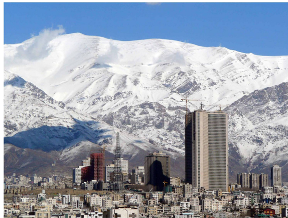
Fig. 3. A Retrofitted 56-Story reinforced concrete building.
