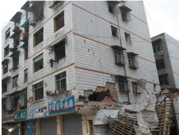
Fig. 1.2 Infill damage after Wenchuan, China 2008 earthquake (Mosalam and Sitar 2008).
