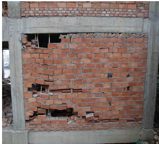
Fig. 1.1 Infill damage after Wenchuan, China 2008 earthquake (Li et al. 2008).
