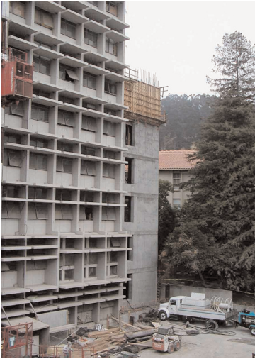
ABOVE: View of west tube under construction.
