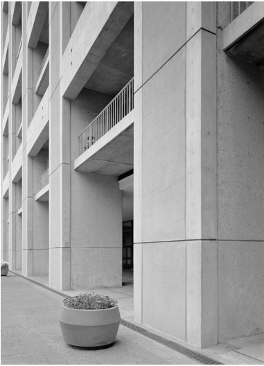
LEFT: Detail of box columns.
