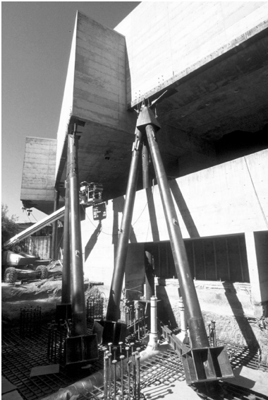
LEFT: Installation of exterior steel columns.
