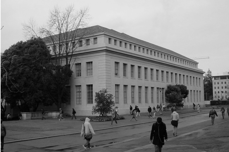
ABOVE: View of Doe Library Annex. Photo courtesy of UC Berkeley Capital Projects.
