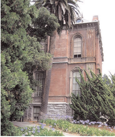
ABOVE: Side view of South Hall.
