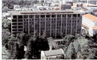
ABOVE: Barrows Hall before retrofit. Photo by Steven Brooks.
