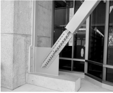
LEFT: Detail of unbonded brace.
