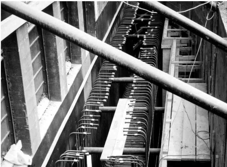
ABOVE: Rebar for exterior shear walls. BELOW: Rebar for foundation.
