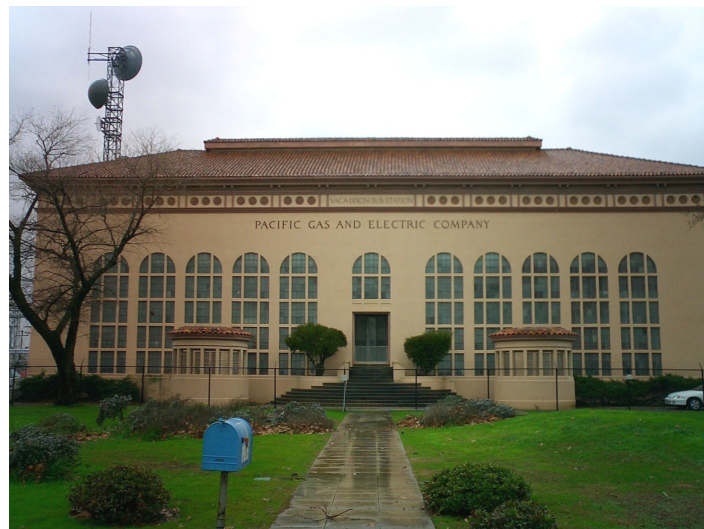
Figure 6.9 One-story mill building with two-story rear portion (R&C 2005a)
