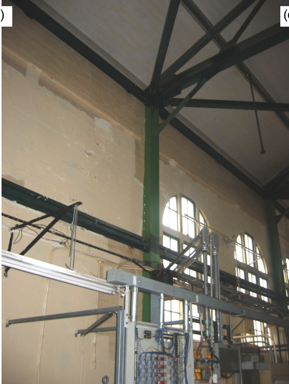
Figure 4.2 Photos of the building: (a) exterior; (b) interior showing existing steel framing, added horizontal steel beam for wall out-of-plane support, and added steel members for roof diaphragm bracing; (c) close up of existing steel column made up of four angles riveted to a web plate.
