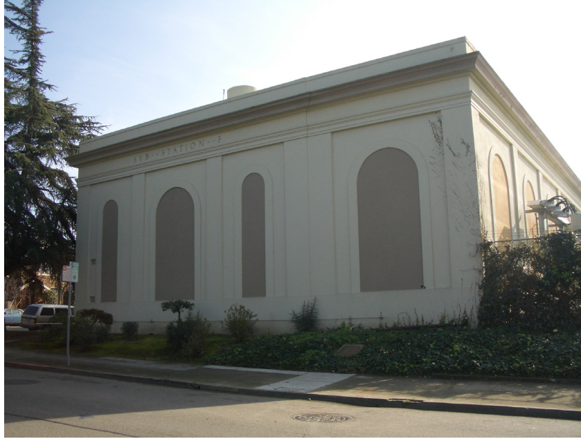
Figure 6.17 One-story mill building with flat roof and skylights (R&C 2006b)
