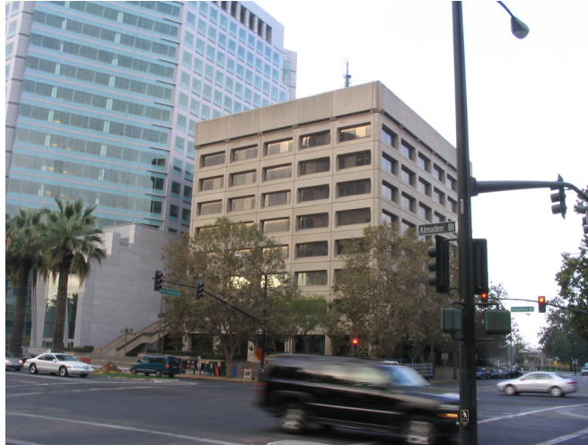
Figure 6.1 Eight-story moment-frame building (R&C, SGH 2004)
