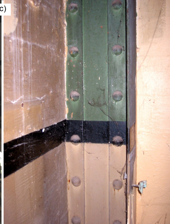
Figure 4.2 Photos of the building: (a) exterior; (b) interior showing existing steel framing, added horizontal steel beam for wall out-of-plane support, and added steel members for roof diaphragm bracing; (c) close up of existing steel column made up of four angles riveted to a web plate.
