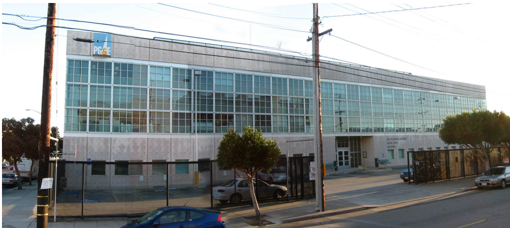
Figure 2.1 Photo of the building exterior
