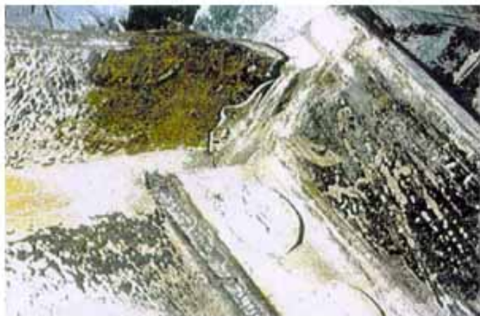
Figure 4.2.4 Crack in Top Flange of Beam, 1R
