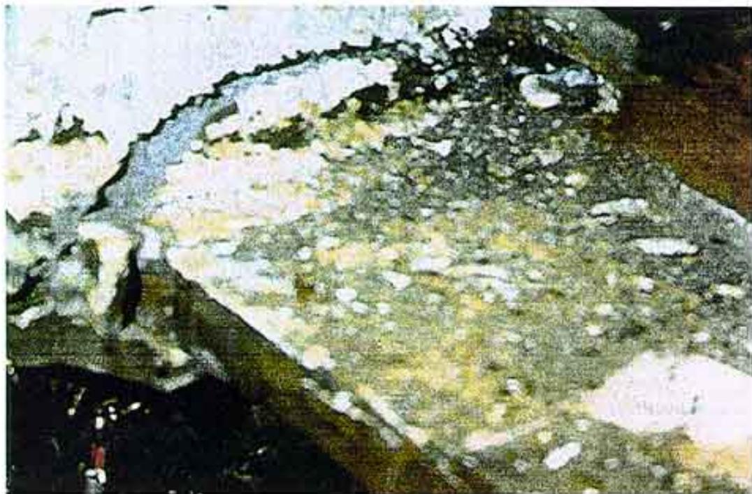
Figure 4.3.3 Pullout at Bottom Flange of Beam
