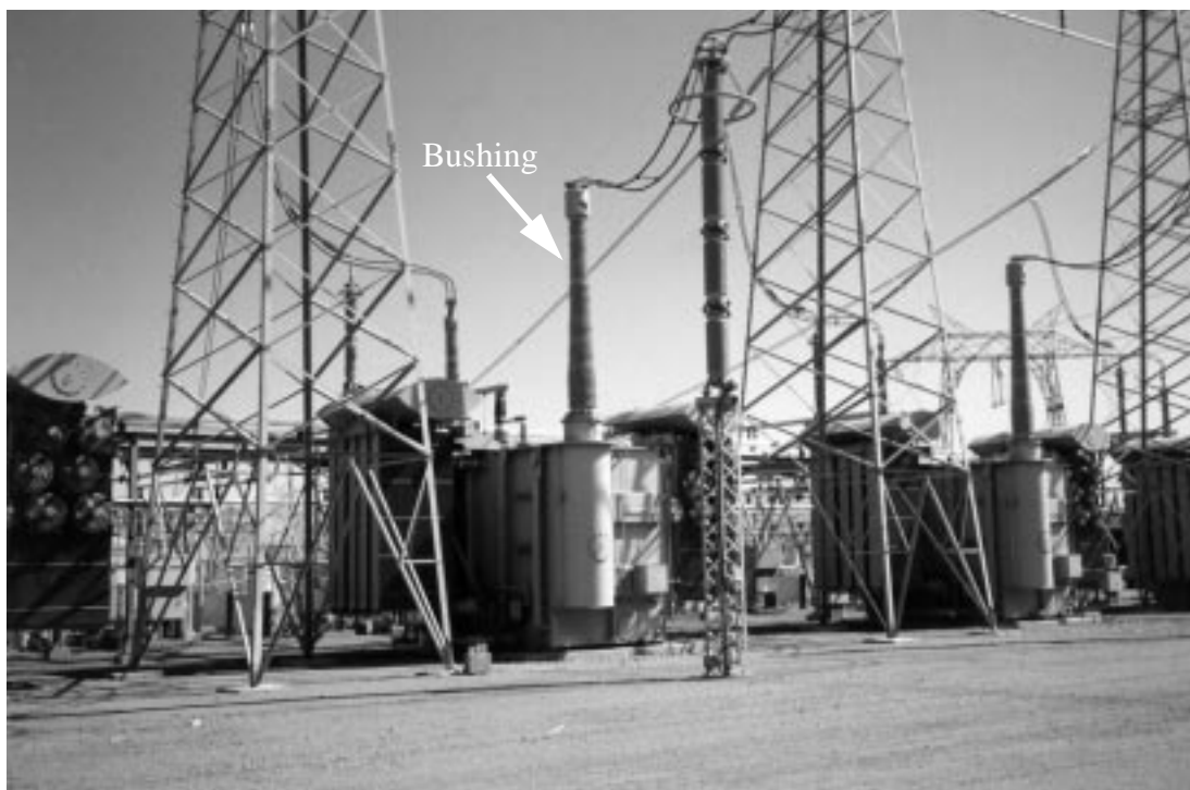
Figure 1-1 Photograph of a bushing mounted on an oil-filled transformer
