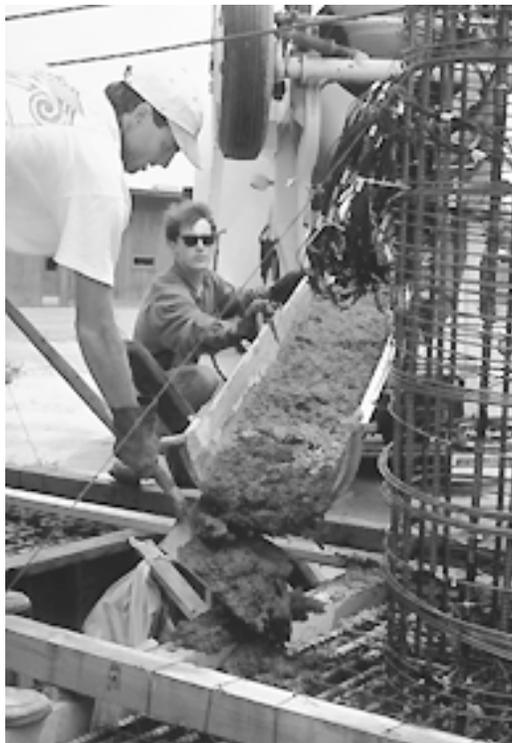
**Figure A.15: Casting Anchor Blocks**
