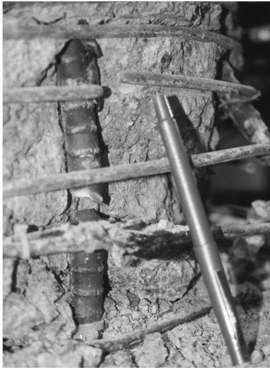
**Figure 3.12: Column 407 Fractured Main Longitudinal Bars**
