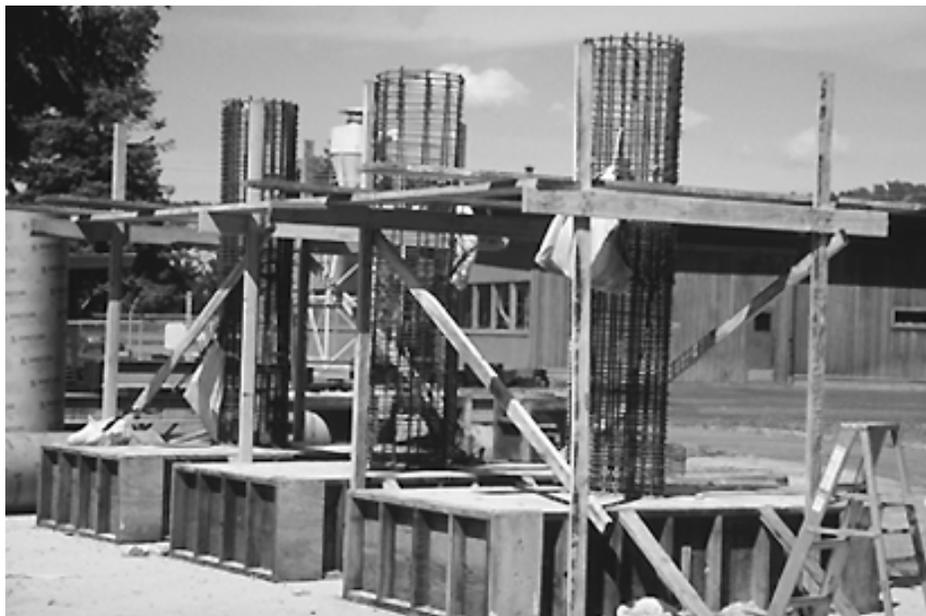
**Figure A.12: Three Columns of Test Series I after Casting Anchor Blocks**
