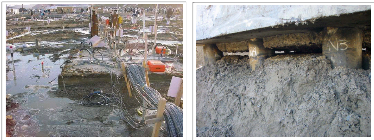
Figure 42. Settlement and expelled pore water near the 9-pile group (left) and underside of pile cap (right) after the 1st liquefaction event (from Ashford & Juirnarongrit, 2002 [63])
