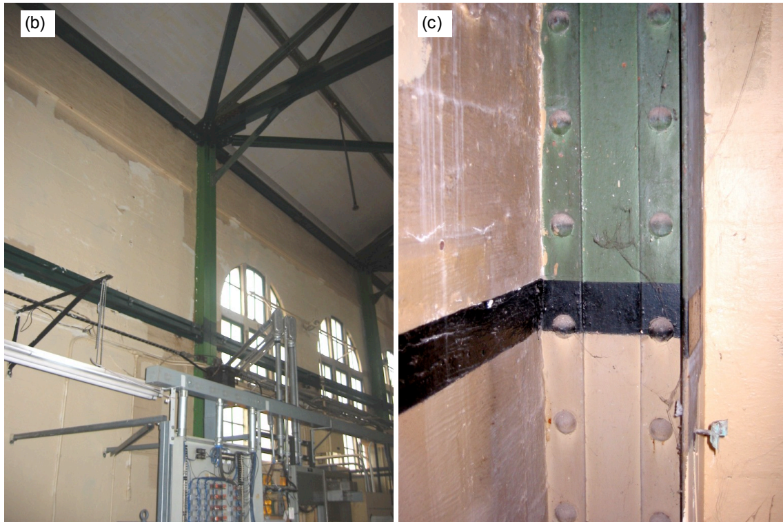
Figure 4-2: Photos of the building: (a) Exterior. (b) Interior showing existing steel framing, added horizontal steel beam for wall out-of-plane support, and added steel members for roof diaphragm bracing. (c) Close up of existing steel column made up of four angles riveted to a web plate
