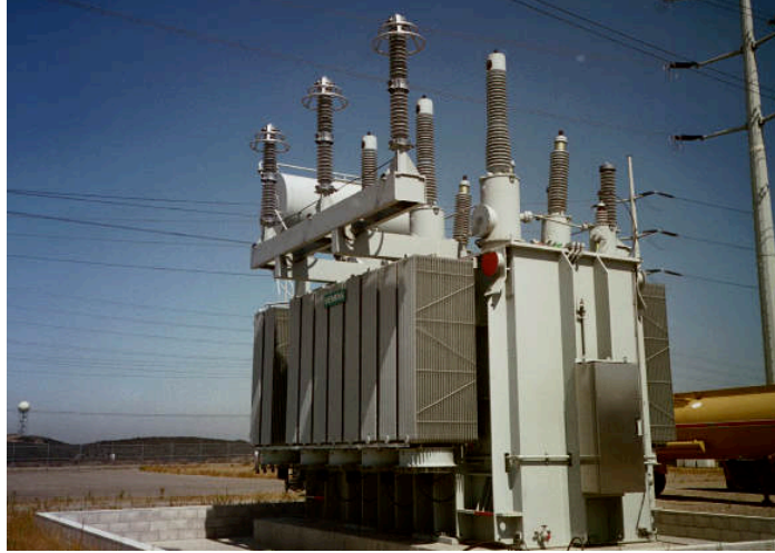
Figure 1.2 - 230 kV Transformer.
