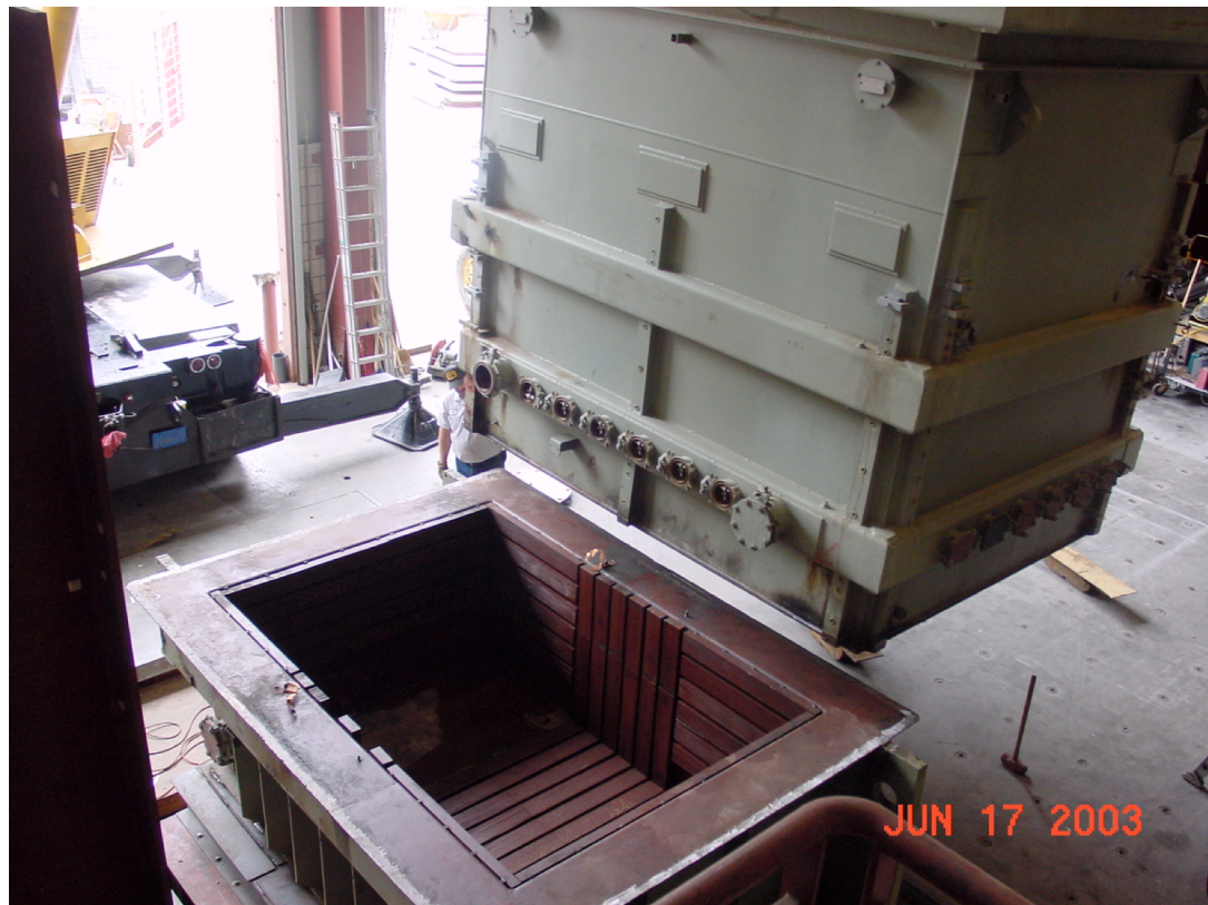
Figure 5.5 - Transformer Test Specimen Being Assembled on Shake Table.
