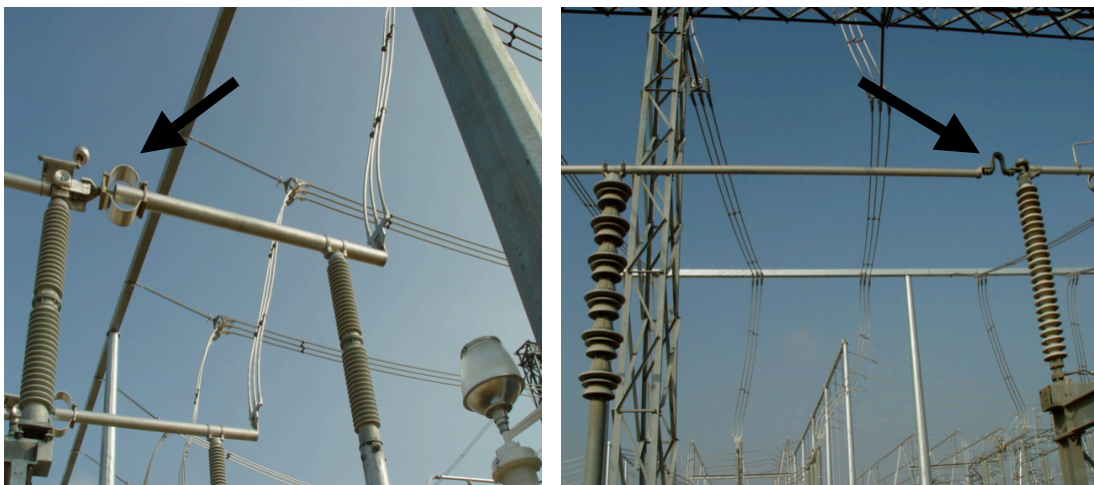
Figure 1.1 Typical Rigid Bus Connectors
