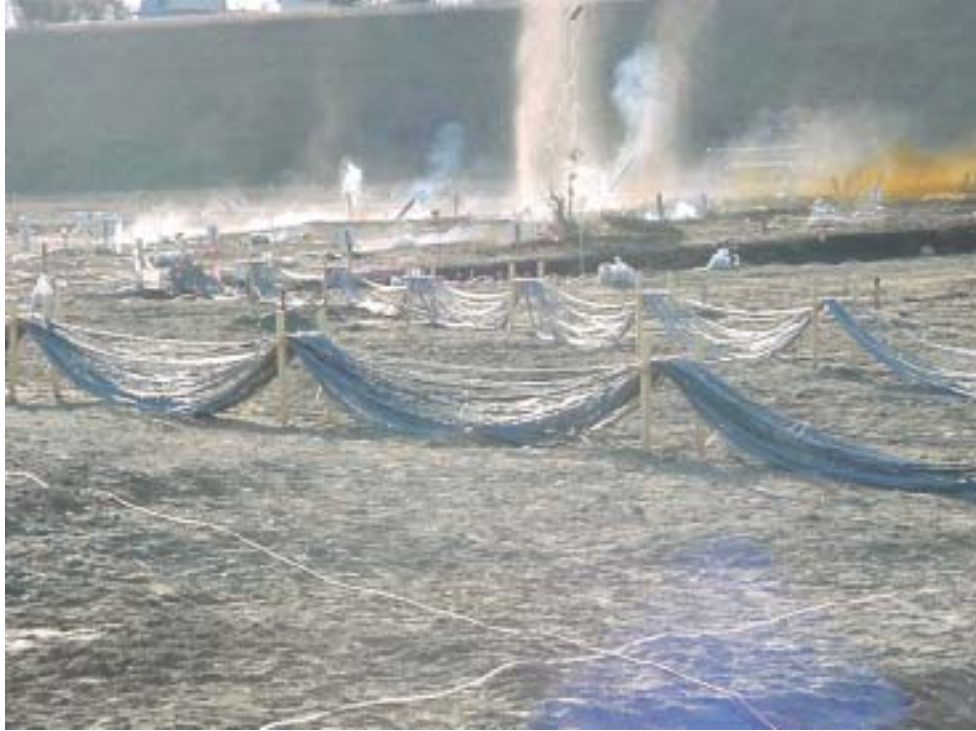
Figure 30 – Blasting underway, November Test
