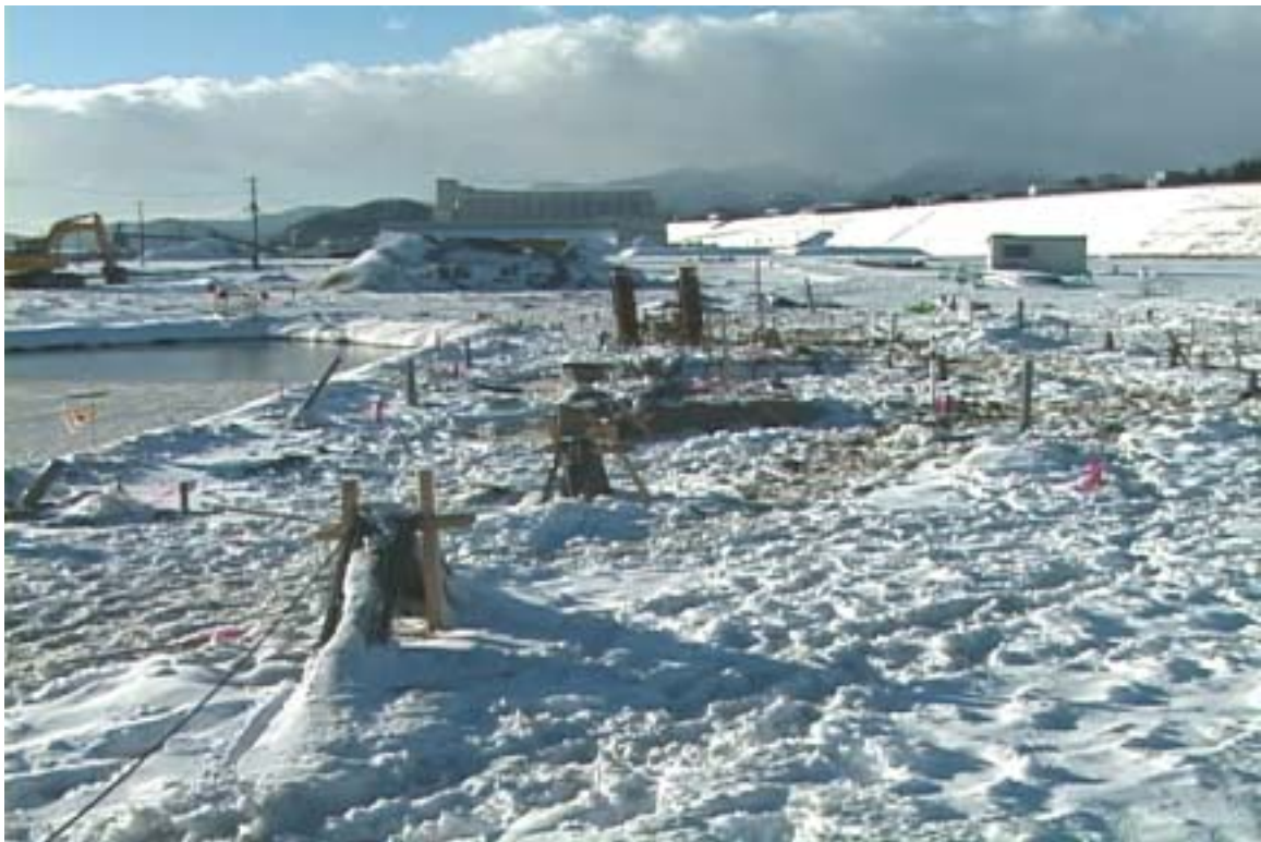
Figure 4 – December 2001 test site.
