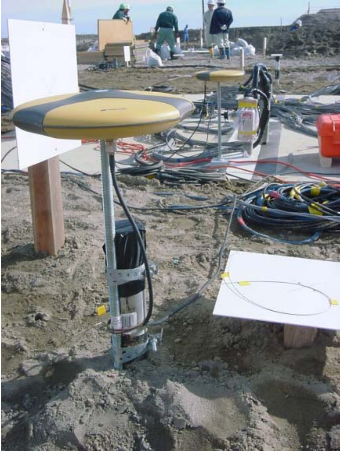
Figure 11 – Units 1A and 1B, November Test
