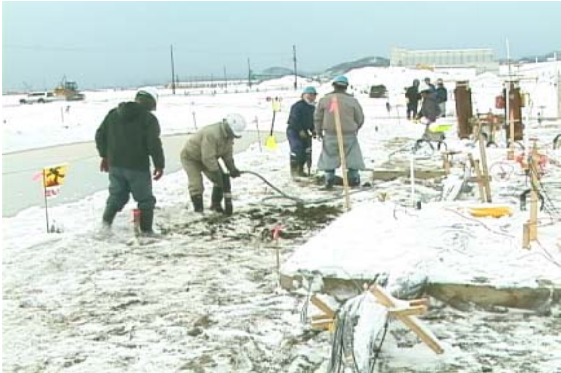
Figure 33 – Jackhammer operation to break up frozen soil surface
