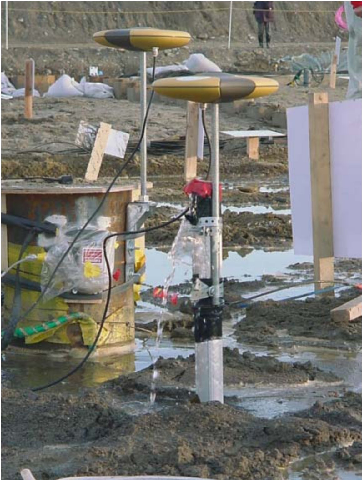
Figure 56 – GPS Units 1D and 1E shortly after blasting
