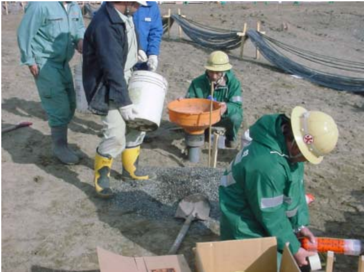
Figure 28 – Placing explosives
