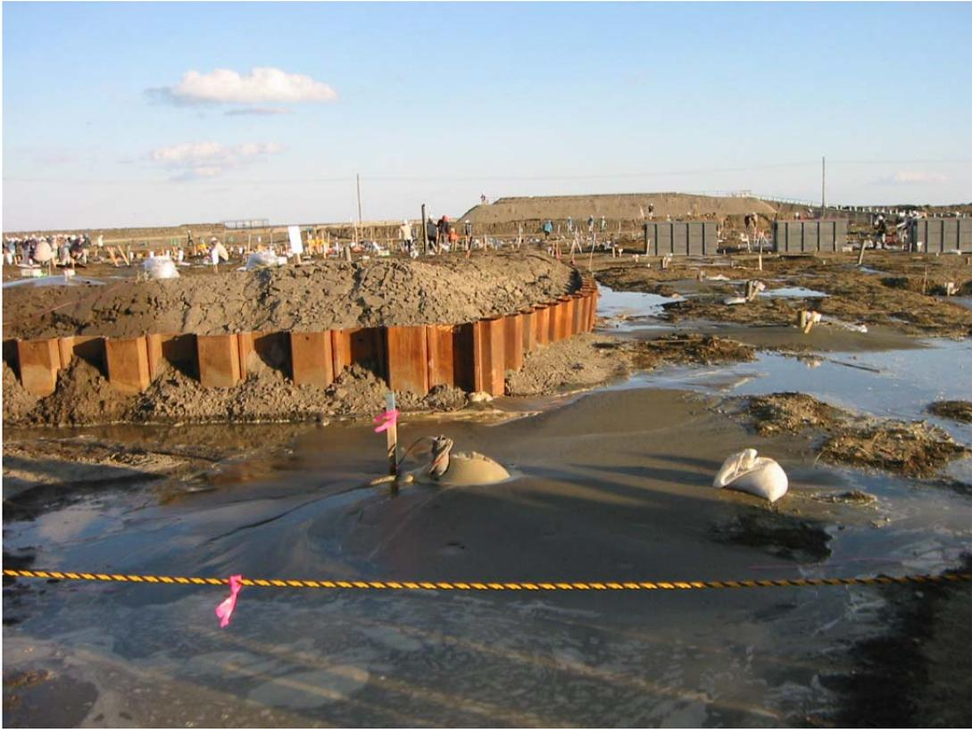
Figure 4.58 Lateral Movement of Sheet Pile due to Effect of Blasting
