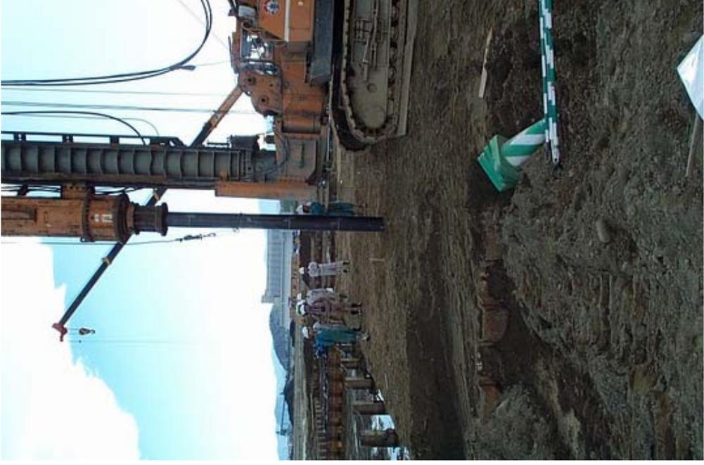
Figure 3.7 Installation of Pile a) Locating Pile to Specified Location , and b) During Pile Driving
