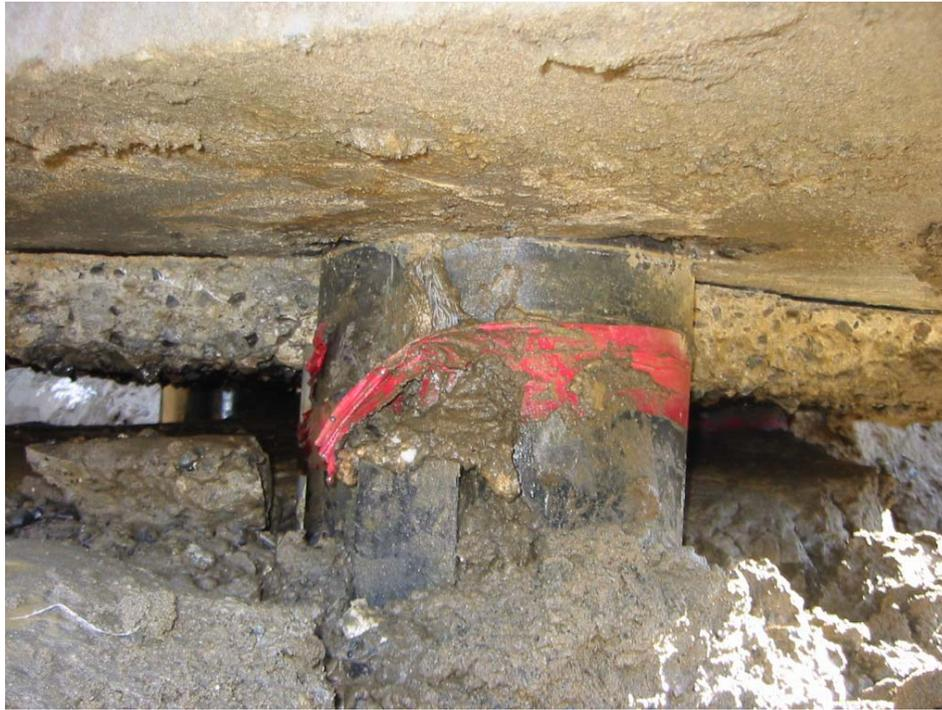
Figure 5.91 Condition of Piles to Pile Cap Connection of 4-Pile Group after Lateral Spread
