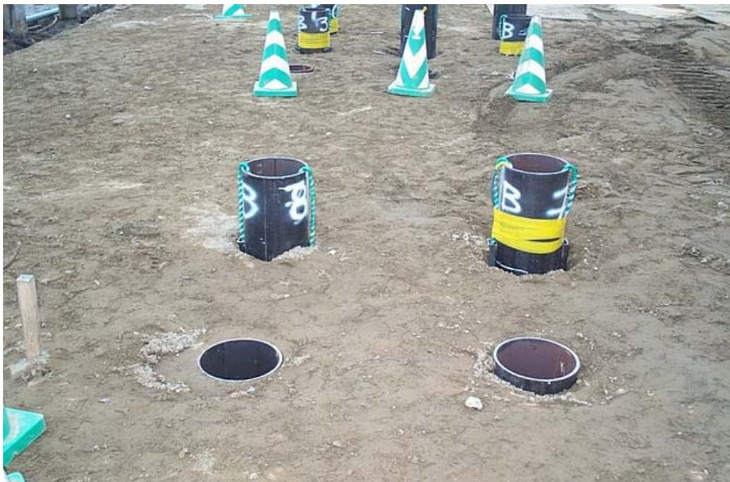
Figure 3.9 Piles of 4-Pile Group after Completion of Installation
