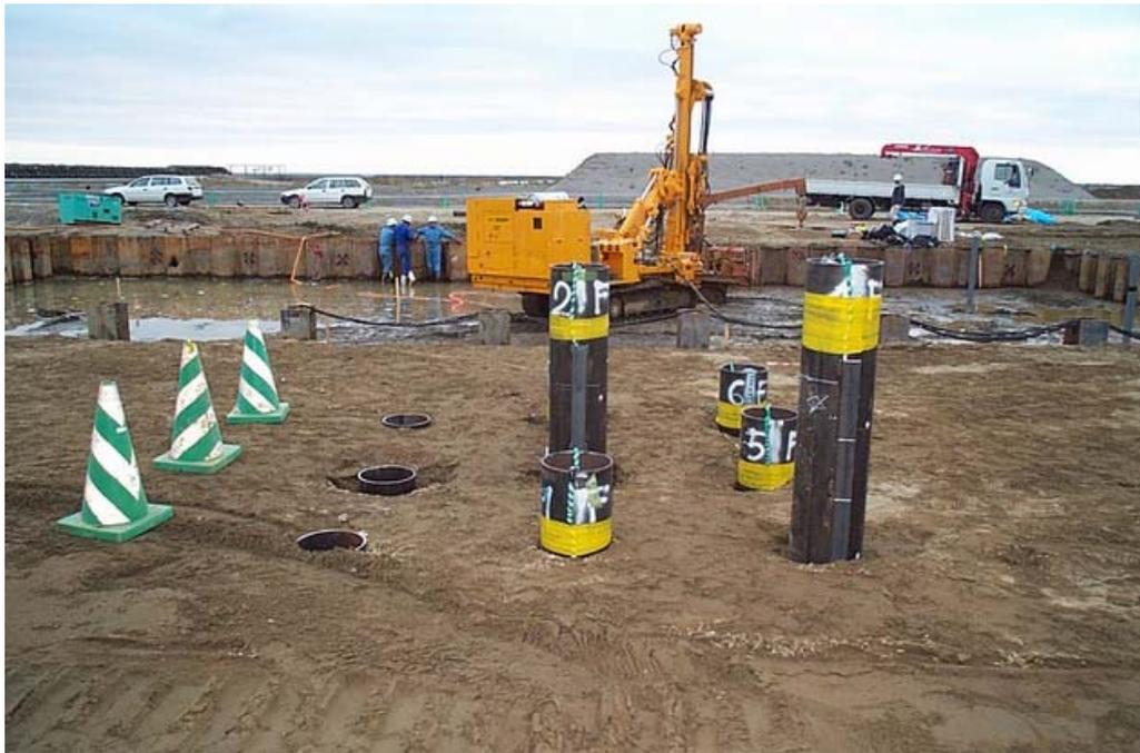
Figure 3.8 Piles of 9-Pile Group after Completion of Installation
