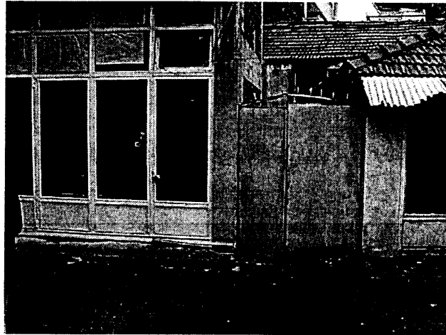
Figure 5-9b: Buckled gate in the back of building B5 evidencing earthquake induced lateral translation of the structure (08/25/1999)
