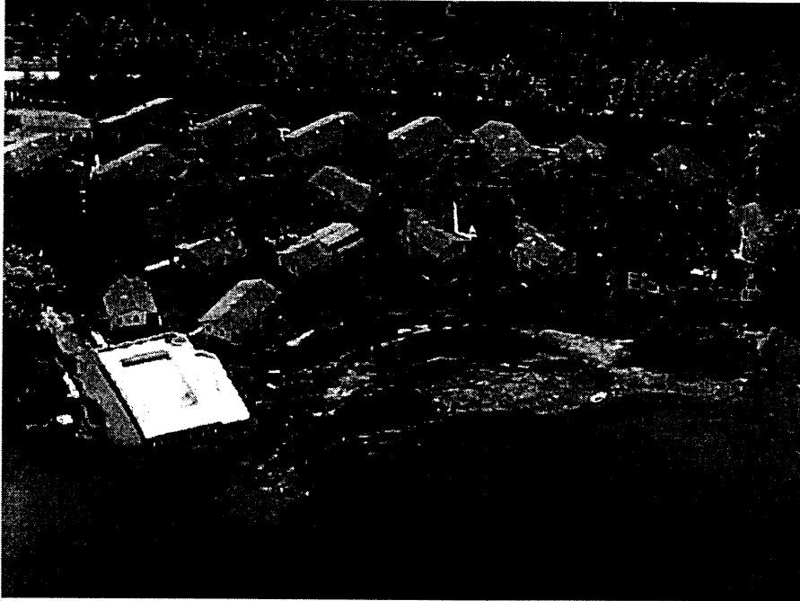
Figure 5-60: Photos taken from the air indicate that a significant zone of subsidence and lateral movement occurred along the coast of Lake Sapanca.
