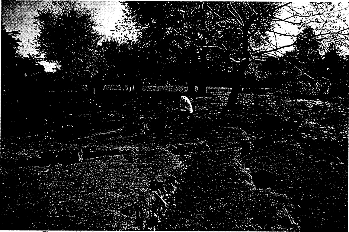
Figure 5-69: View of the police station site that underwent lateral spreading
