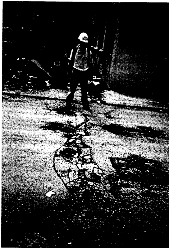
Figure 5-84: Buckling of the pavement in Yakin Street
