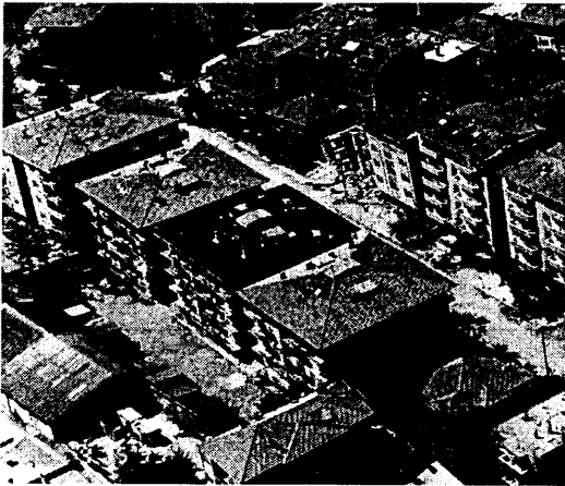
Figure 5-10a: North to south aerial view of Site C before building C1 was demolished. (Photo courtesy of I. M. Idriss)
