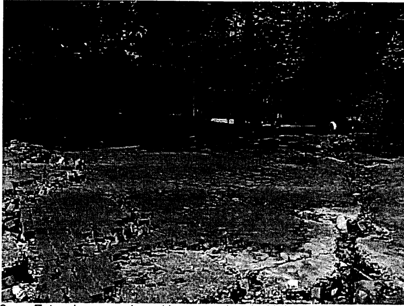
Figure 5-56: Extensive ground cracking, associated with lateral spreading, was observed throughout the grounds of Hotel Sapanca. Generally, these cracks were associated with soil venting.
