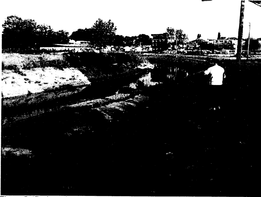
Figure 5-47: A north to south view of the canalized river (Photo by Brady Cox)
