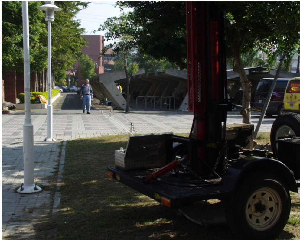
Figure 15.2 Picture Taken at Yuan-Lin Elementary School (View # 1)
