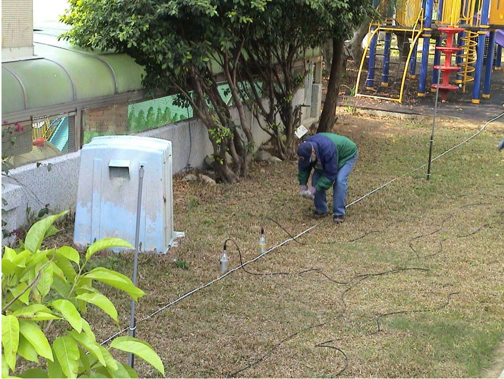
Figure 5.3 Picture Taken at Si-Kon Elementary School (View # 2)
