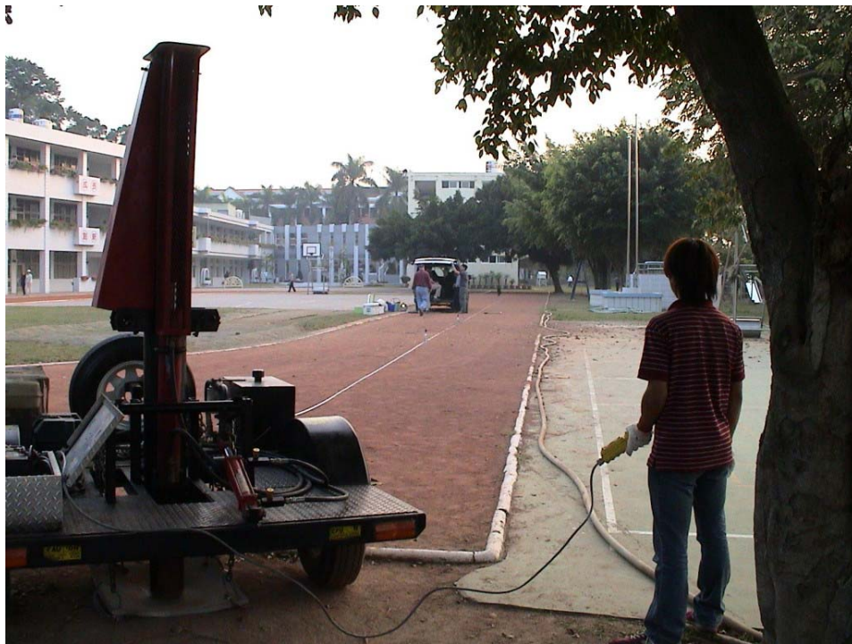
Figure 1.2 Picture Taken at Lin-Chong Elementary School (View # 1)
