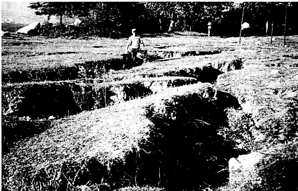
Figure 2.42 Photograph showing the large ground cracking that occurred at Police Station during the earthquake. The surface fault rupture exits the bay near here.
