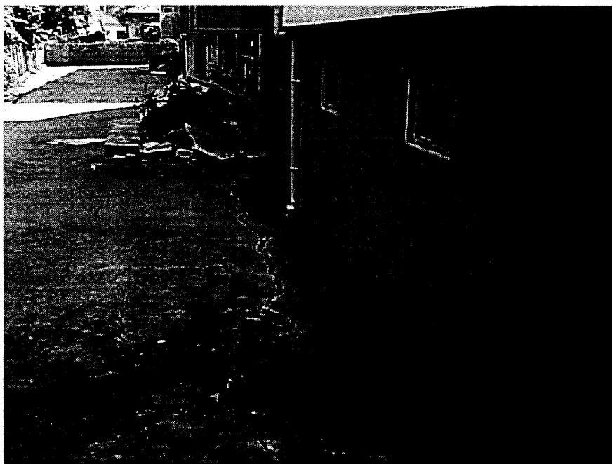
Figure 2.20 Photograph showing the liquefaction-induced settlement at Site J. Notice the liquefaction ejecta (from http://peer.berkeley.edu/turkey/adapazari ).
