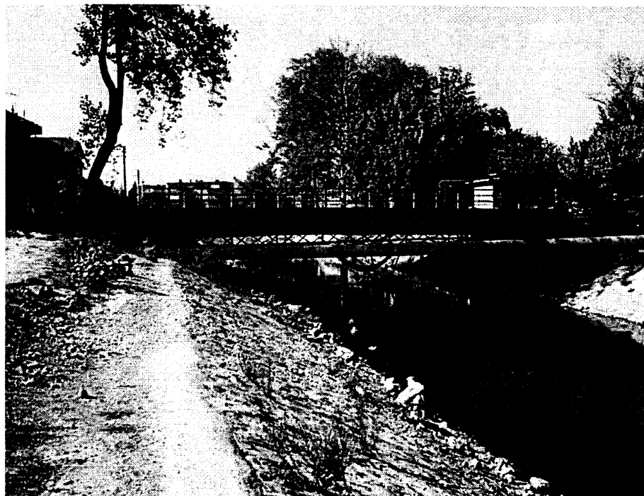
Figure 2.26 Photograph of Site 1-24. No lateral movements were noticed here along the banks of the Çark Canal.
