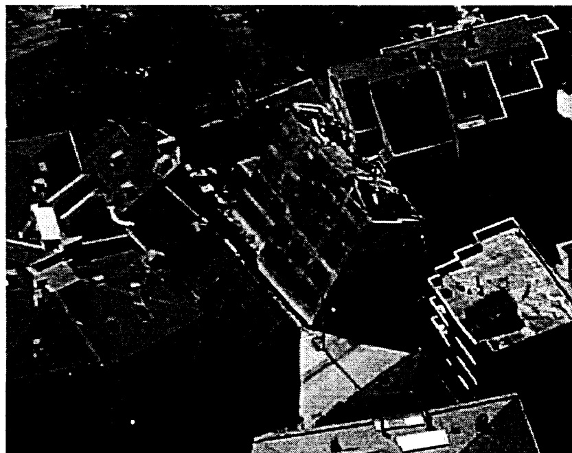
Figure 2.17 Photograph of Site G, where liquefaction of foundation soil caused buildings G2 (right) and G3 (left) to tip apart in a "V" (from http://peer.berkeley.edu/turkey/adapazari ).
