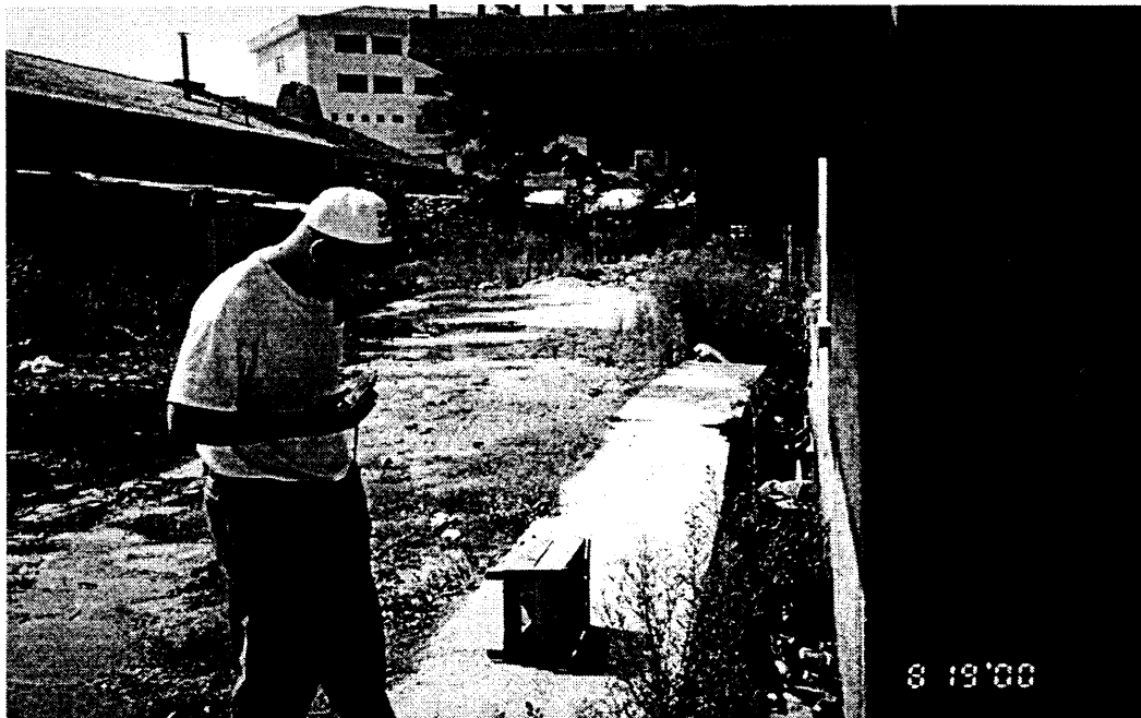
Figure 2.10 Photograph of building C2, which translated 57 cm towards the street (right). Notice the gap between the building and the sidewalk.
