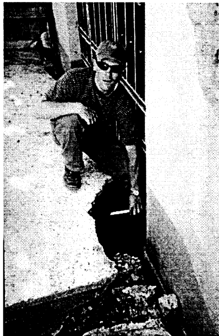
Figure 2.23 Photograph showing approximately 30 cm of settlement between the stairs and the doorway of building N-1 at Site 1-11.
