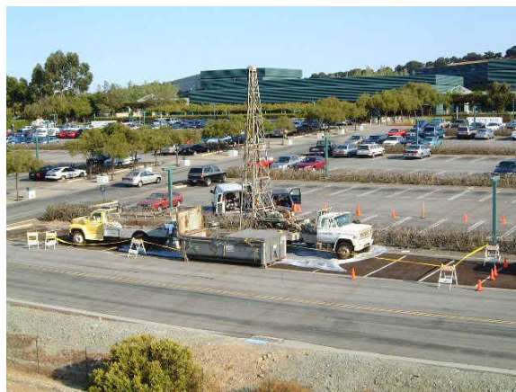
Drill site of IBM Almaden site looking Northeast.
