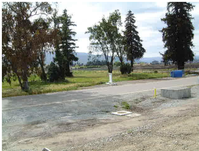
View of Gilroy drilling location.
