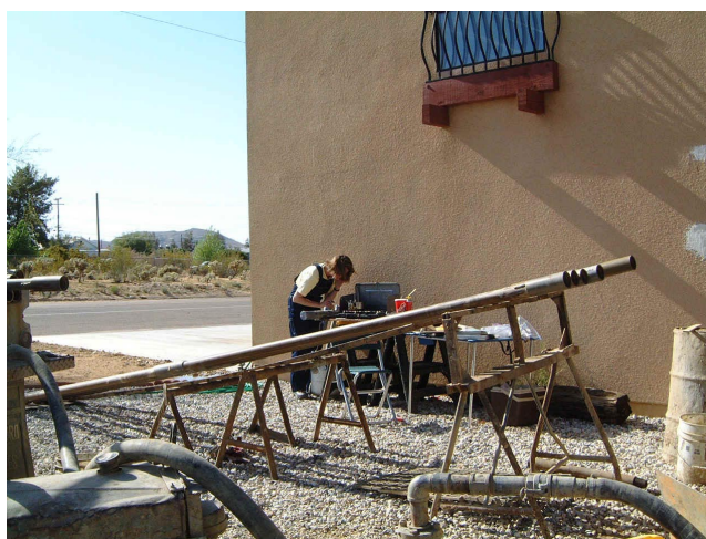
Drilling and sampling activities.
