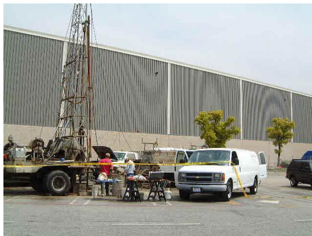
Drill site next to Bell Postal Facility.
