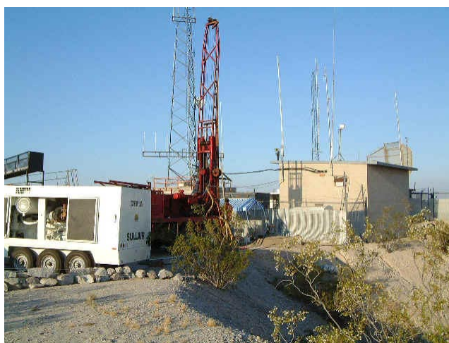
Drill site looking toward the radar station.
