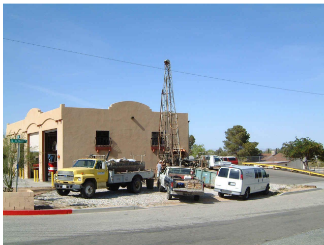
Drill site next to Joshua Tree fire station.
