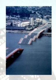
Liquefaction & lateral spreading are a major cause of foundation damage during earthquakes.
