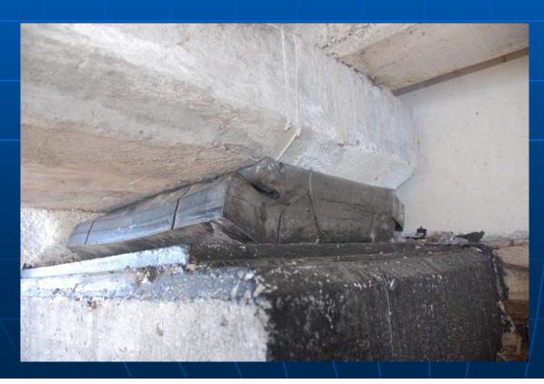
A 15 cm tall 60cm by 60cm elastomeric bearing ruptures due to shear at shear strain of about 70%
