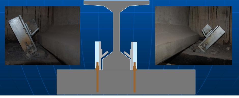
Skewed PC girder bridges recently built without diaphragms and effective side stoppers suffered extensive damage
