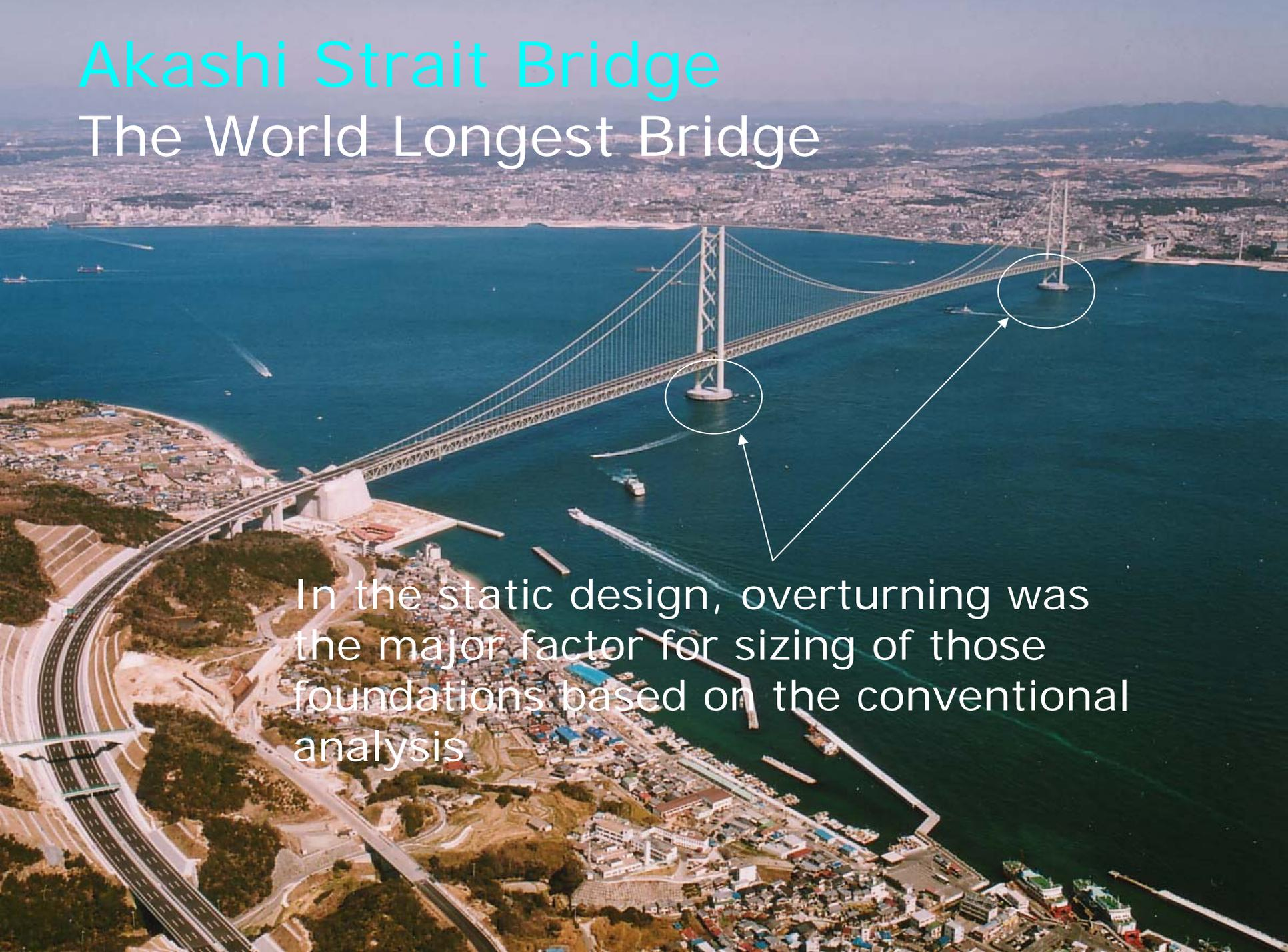
In the static design, overturning was the major factor for sizing of those foundations based on the conventional analysis
