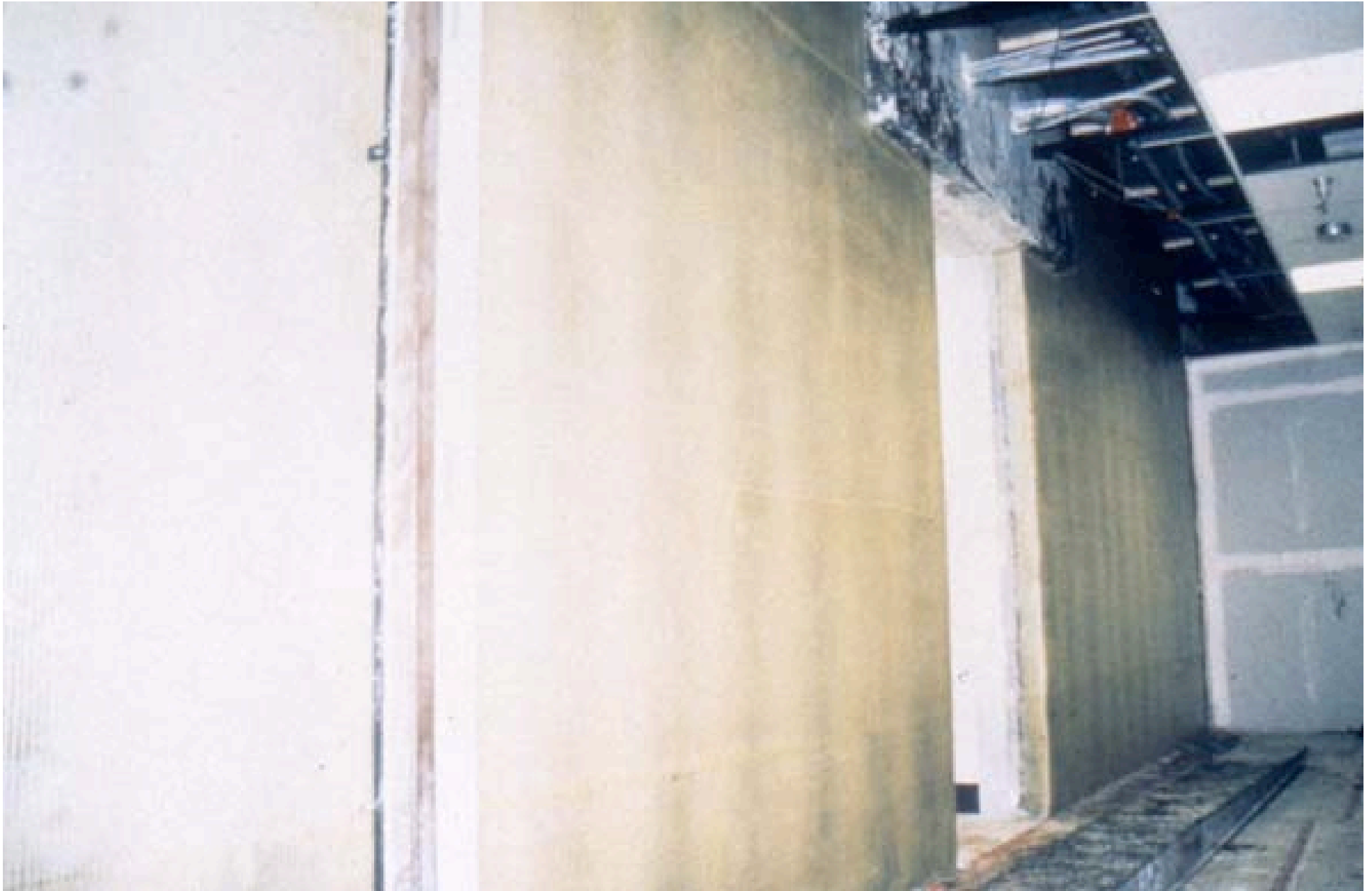
Fiber Overlay Before Finish Plaster
