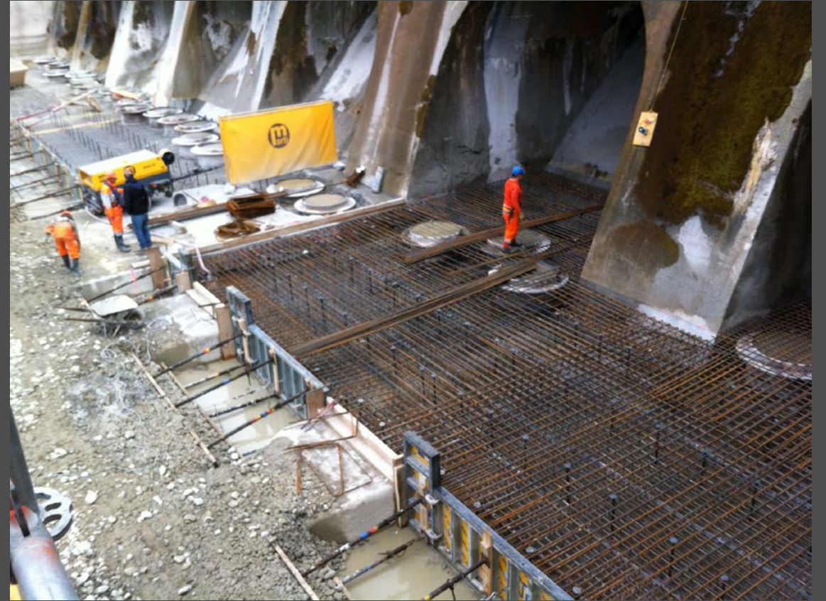
Pile cap steel reinforcement
