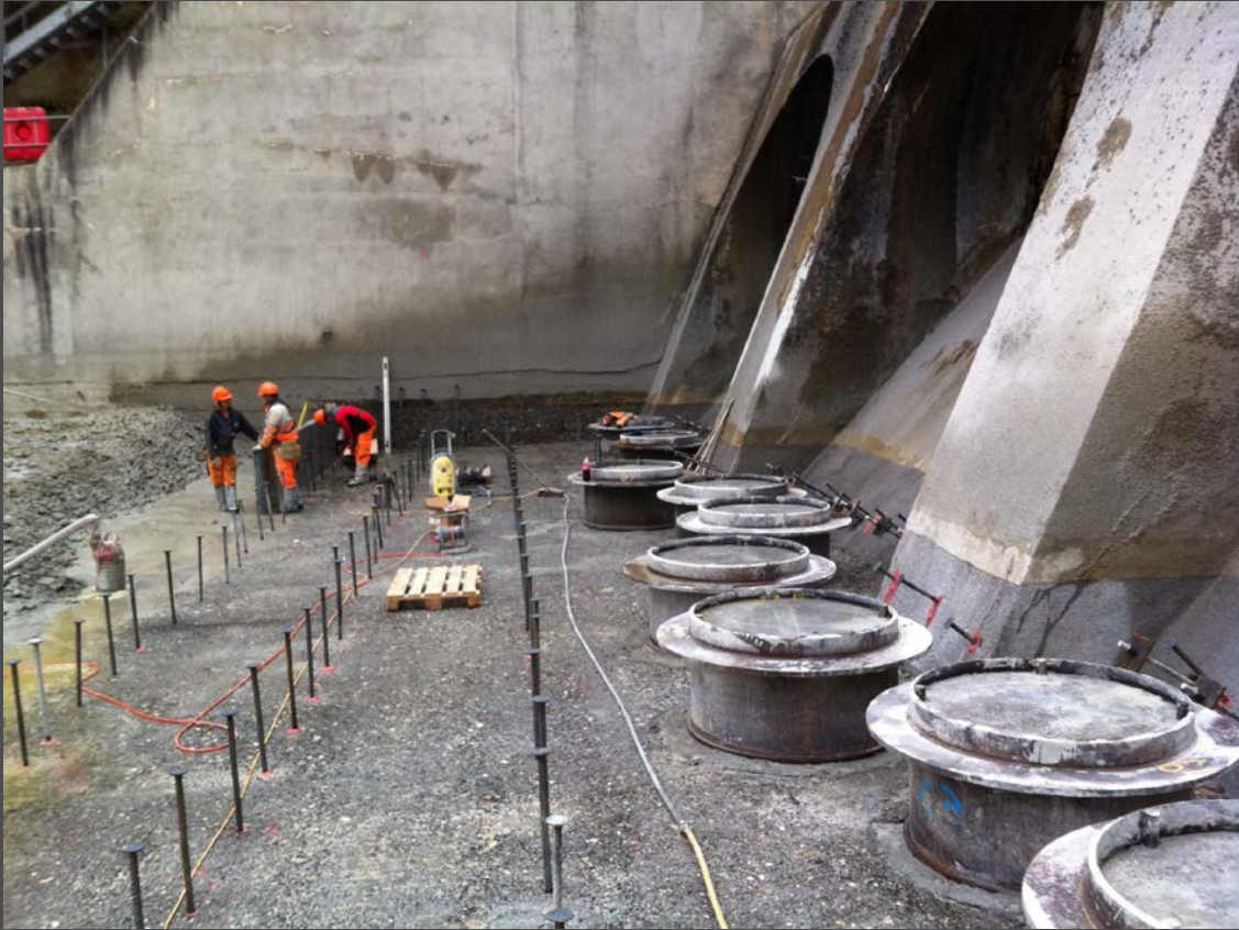
Piles installed at Weir toe
