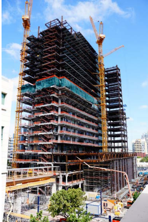
Courthouse under construction (2015)
