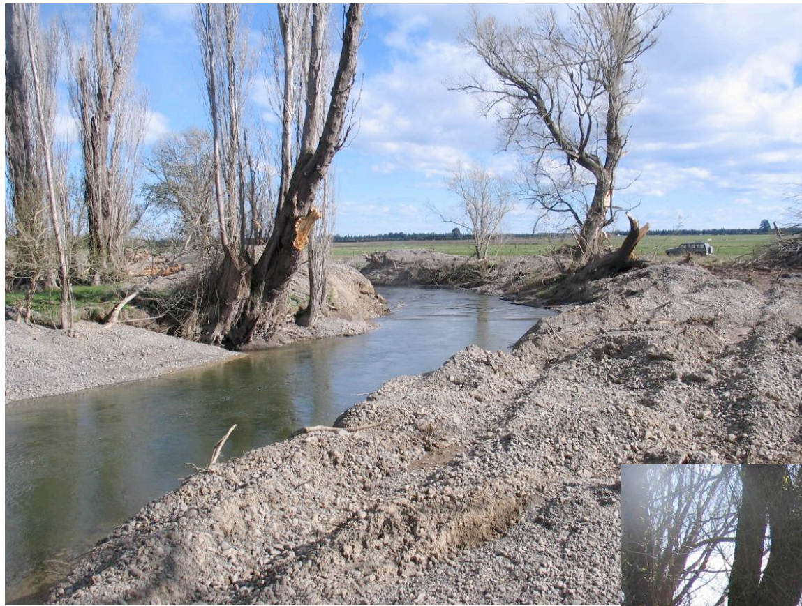
Looking downstream of excavated river bed
