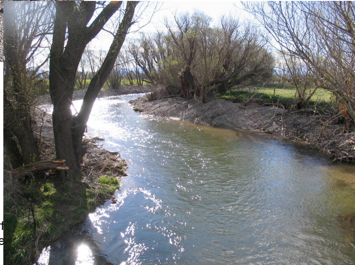
Lower end of excavated river bed, at bridge
