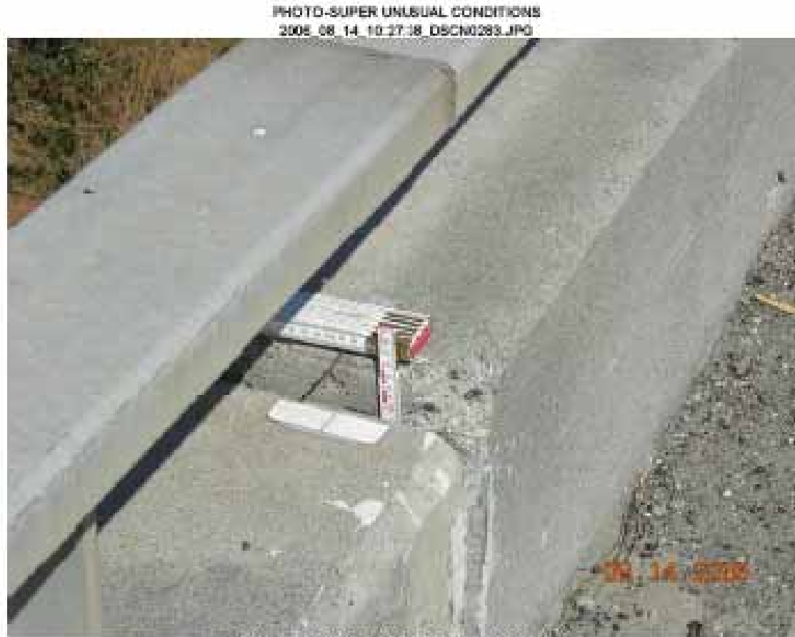
370005L - SARGENT BRIDGE & OH - 04-SCL-101-R.17 Offset in left bridge barrier at second hinge in Span 4.
