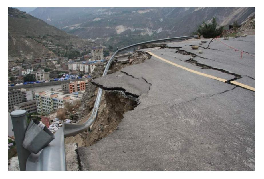
Road damage due to landslide near Yingxiu
