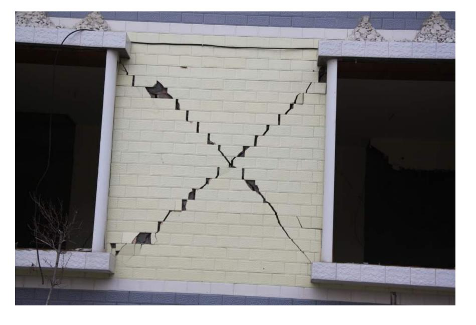
Typical damage for a brick structure
