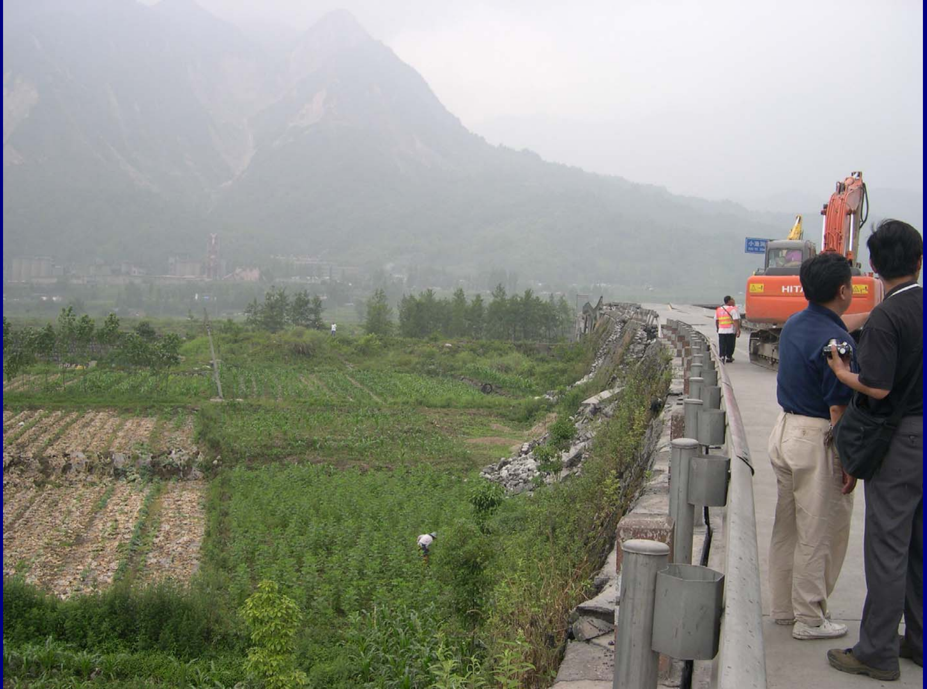
Fault offset near Xiaoyudong bridge (Courtesy of B.G. Zhou of IGCEA)
