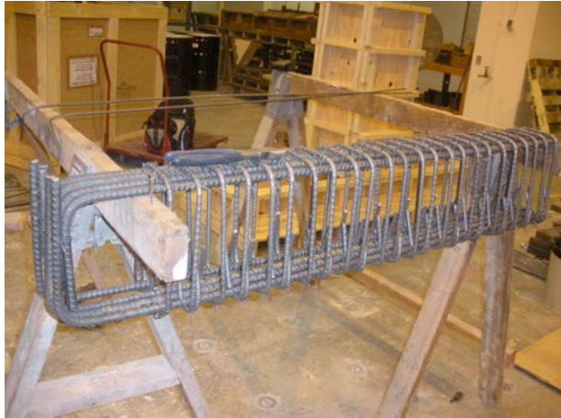
Figure 3.13: Longitudinal beam reinforcement
