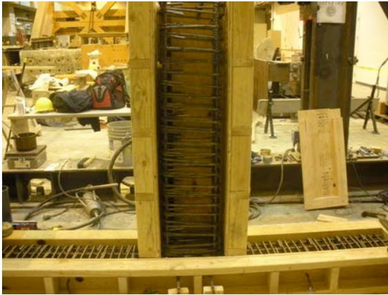
Figure 3.21: Unit before casting
