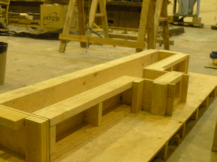
Figure 3.11: Concrete form for the column & transverse beam
