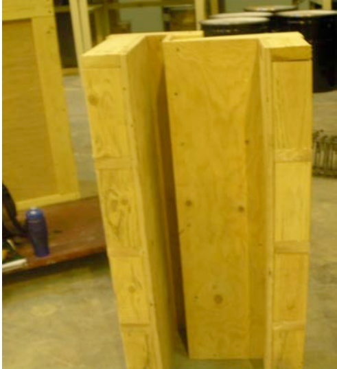
Figure 3.10: Concrete form for the beam
