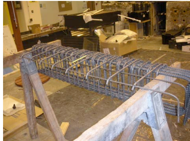
Figure 3.14: Longitudinal beam & slab reinforcement
