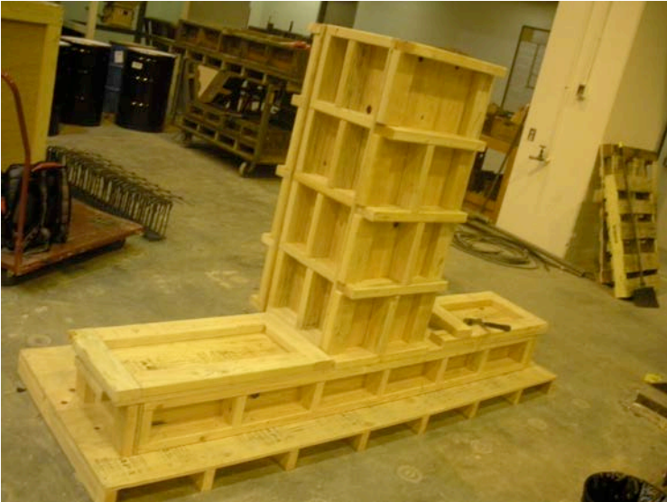
Figure 3.12: Concrete form for the beam column specimen
