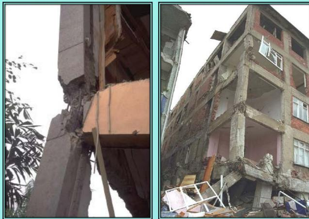
**Figure 1: Non-ductile Beam Column Joint Failure.**
