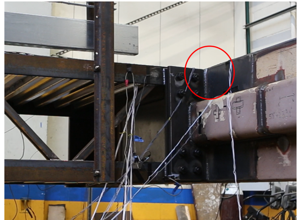
(b) Initial Connection Failure
