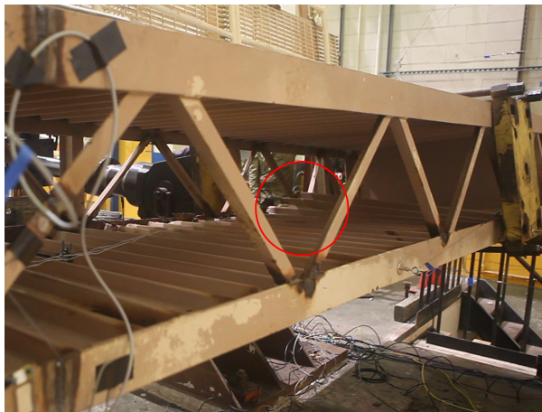
(a) Permanent deformation near actuator (Push direction)
