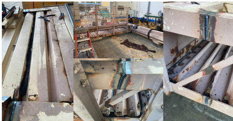
Figure 5.2: Sign Structure after welding
