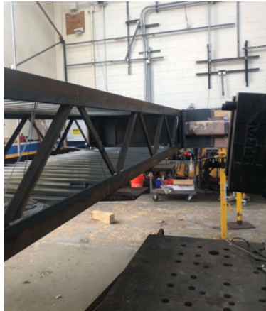
Figure 5.13: Uncorroded Beam Reassembling
