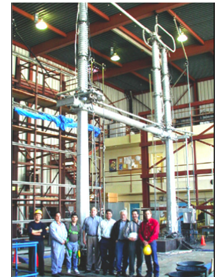
Electrical Equipment Testing (IEEE-693)
