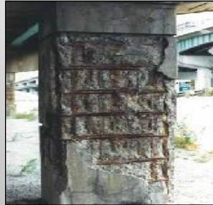
(ASR) Environmental Damage (Corrosion)
