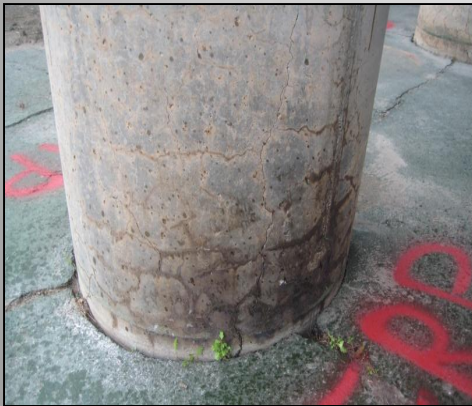
(ASR) Environmental Damage (Corrosion)
