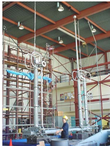
Figure 2 550-kV switch in the open position mounted without the tall supports.
