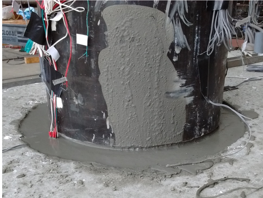
Figure 9 Grouting column-foundation connection
