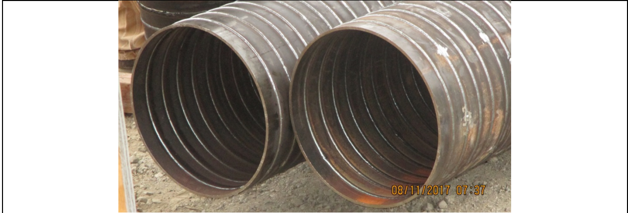
(b) Weld beads at column ends
