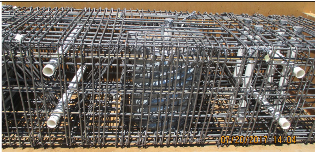
(c) Assembled reinforcement cage, cap beam
