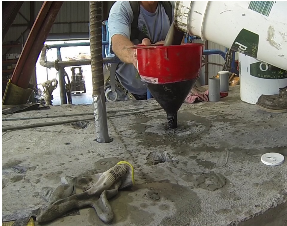
Figure 12 Grouting column-bent-cap connection
