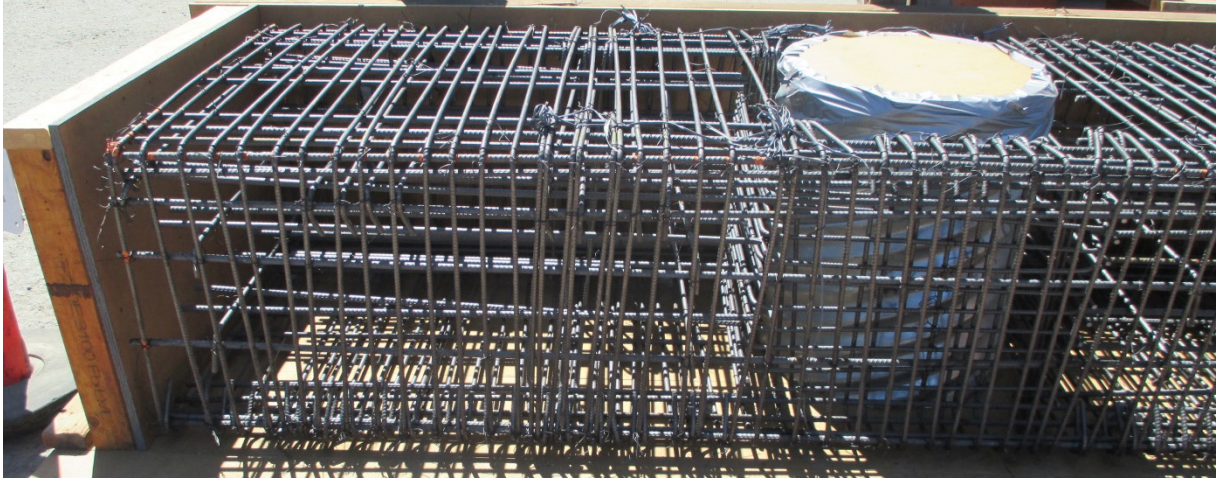
(a) Socket detail in foundation
