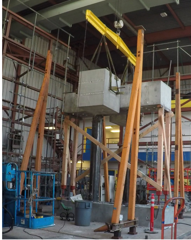
Figure 13 Installation of inertia blocks
