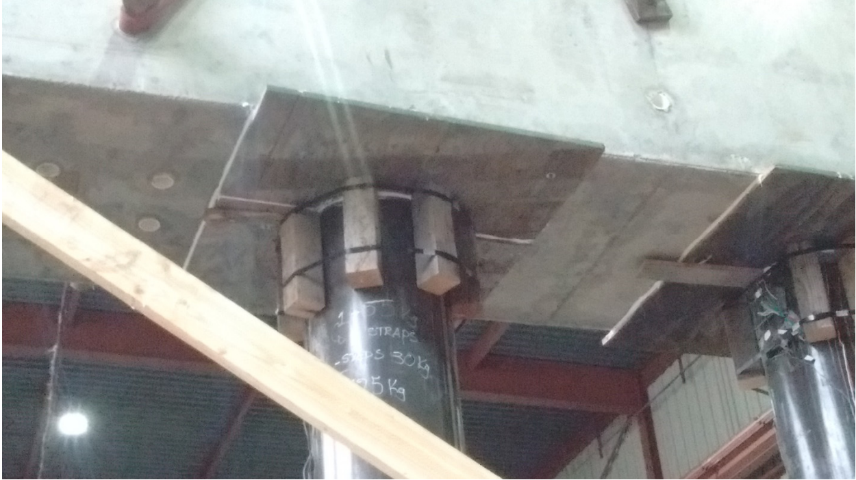
Figure 11 Preparation for grouting the column-cap-beam connection
