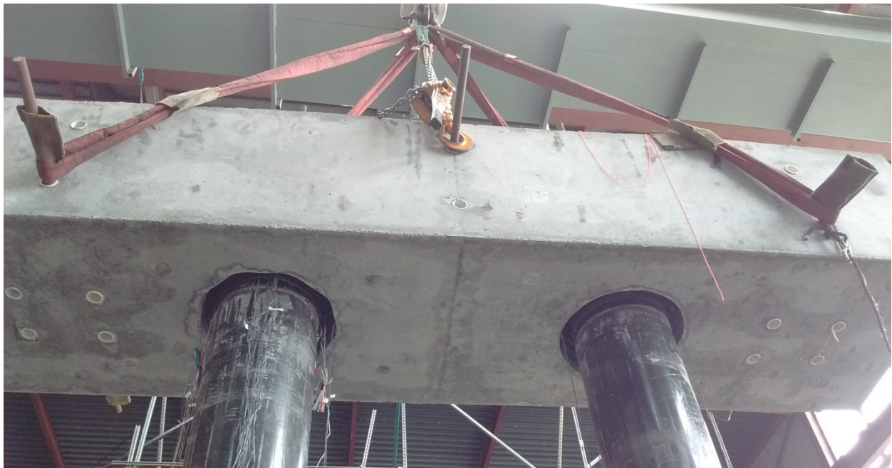
Figure 10 Installation of cap-beam
