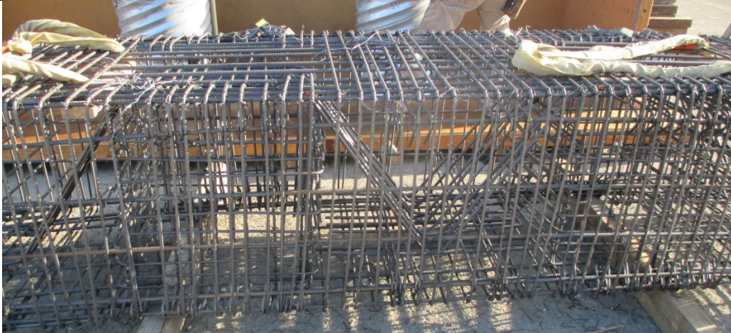
(b) Socket reinforcement detail in cap beam
