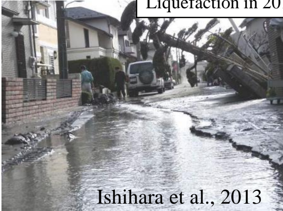
Liquefaction in 2011 Tohoku Earthquake
