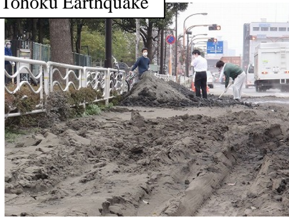
Liquefaction in 2011 Tohoku Earthquake
