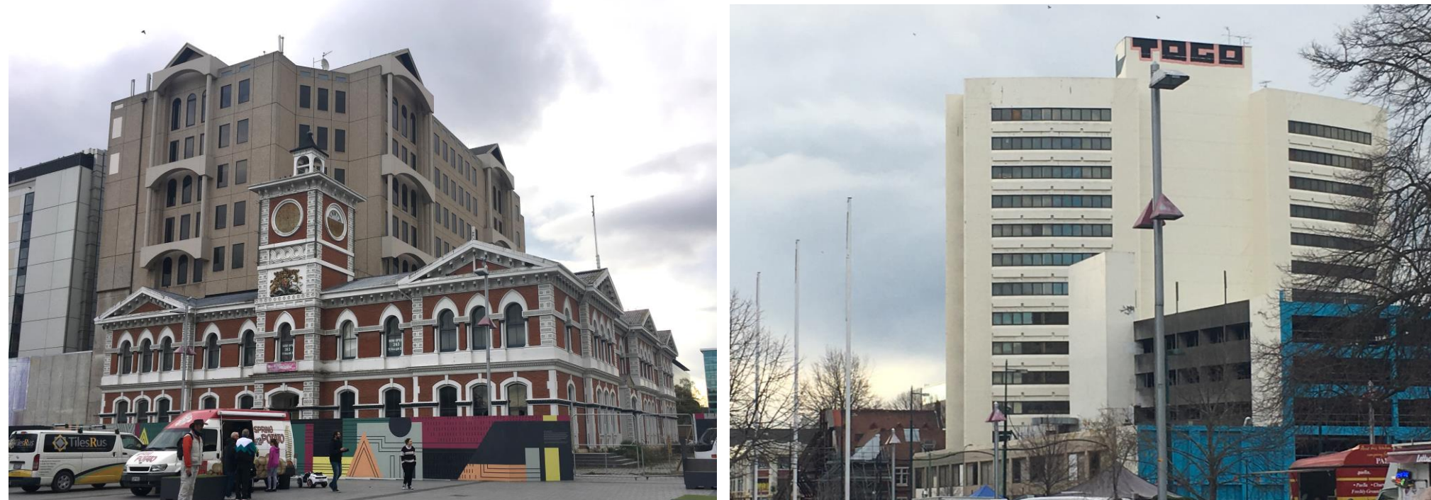
Fig 1. Vacant buildings in Christchurch (September, 2017).
