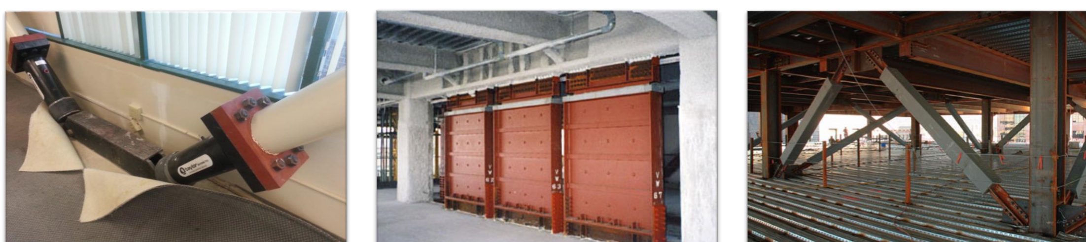
Supplemental energy dissipation devices
