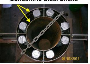
Permanent formwork, replace reinforcing cage, prevent concrete implosion.
