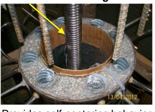
Provides self-centering behavior together with gravity. Threadbar can be easily replaced.
