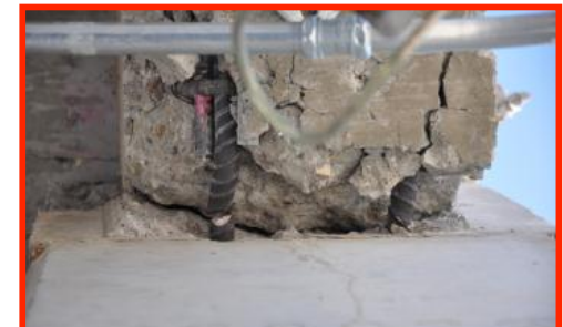
Structural rebar fracture
