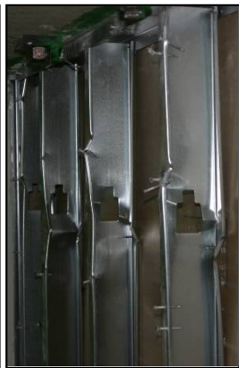
Hinges forming in studs (institutional construction)
