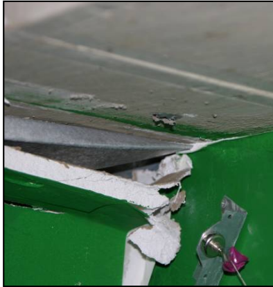
Damage in transverse wall top track
