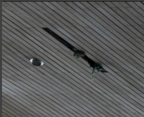
Closeup view of some sprinkler heads sheared off
