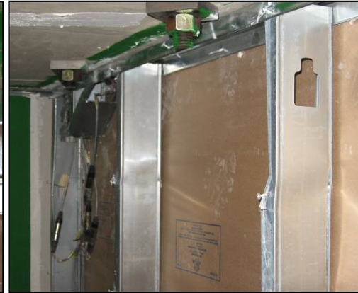
Hinges forming in studs (commercial construction)
