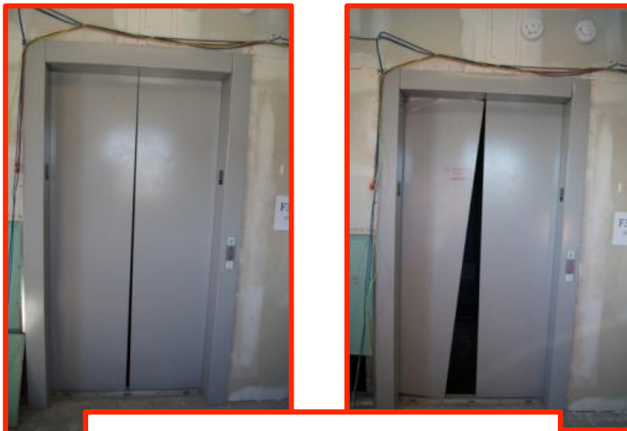
Elevator door distortion
