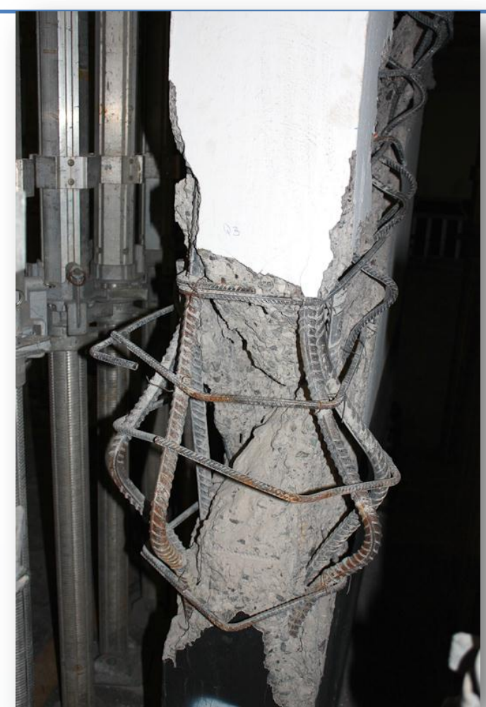
Shear wall boundary element of Chile 2010
