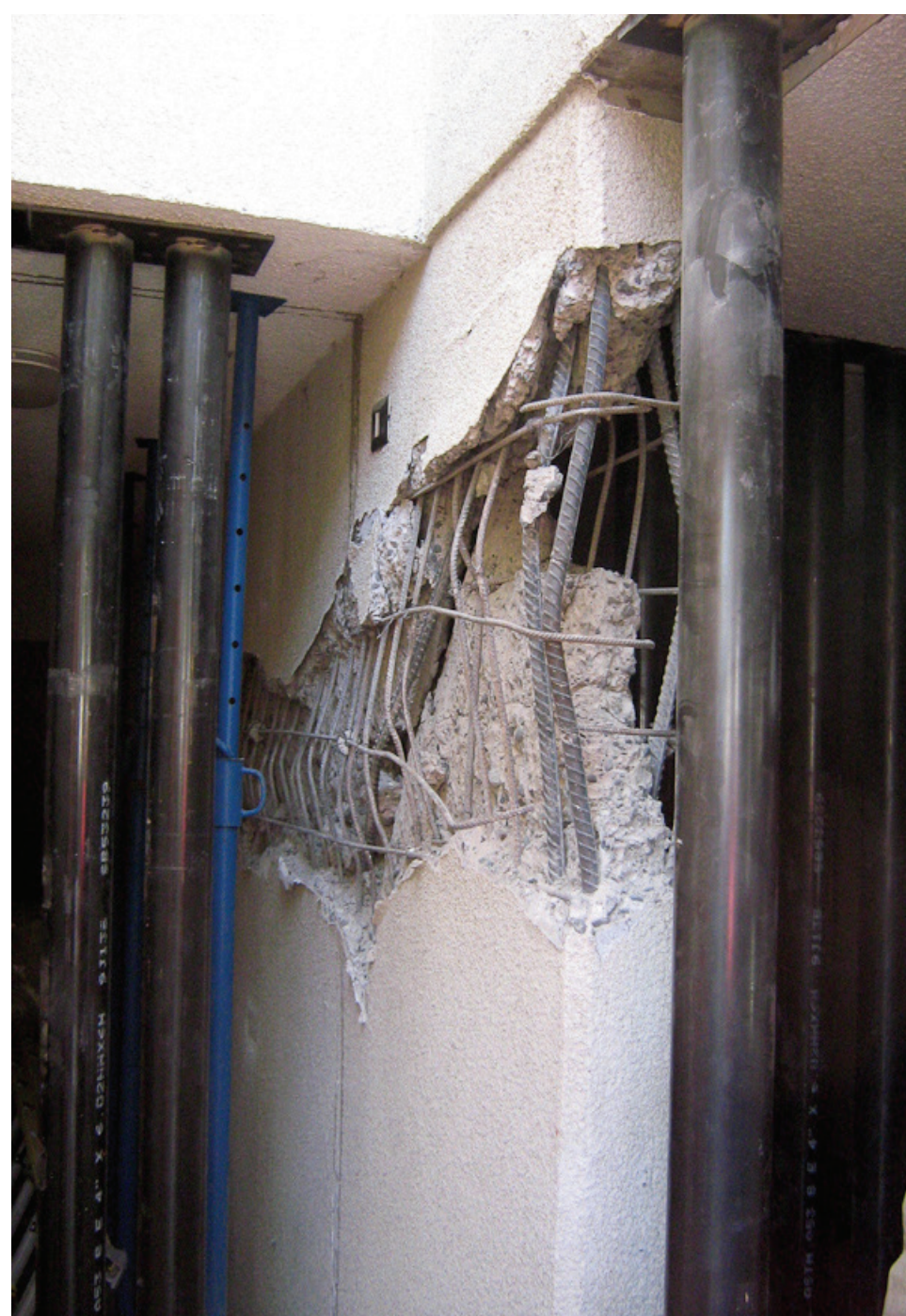
Boundary Element Crushing Failure observed in Chile 2010 Earthquake
