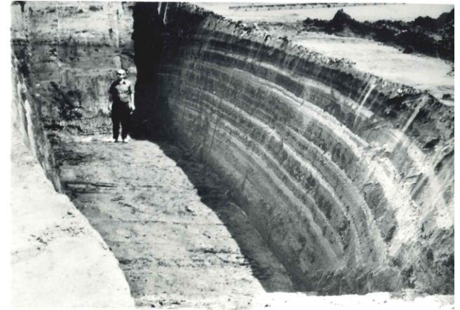
Pronounced layering of dam shell (photo from Upper San Fernando Dam)
