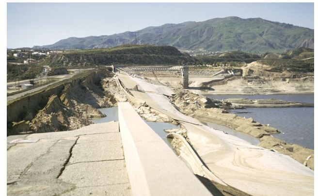
Response of Lower San Fernando Dam (EQIIS, Steinbrugge collection)
