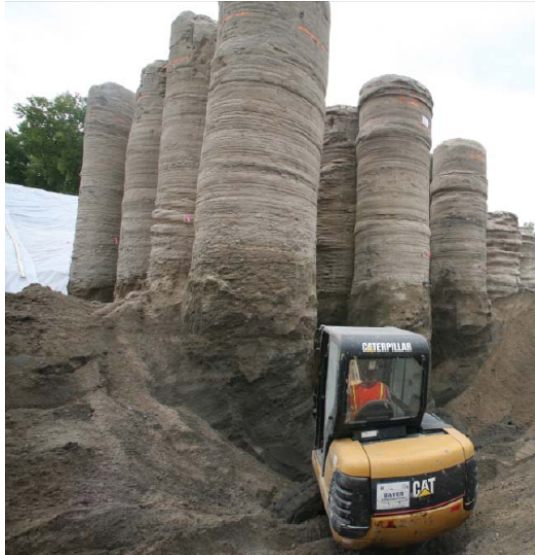
Jet grout columns (John Dillon 2009)
