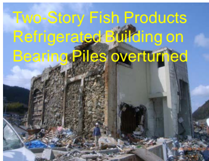
OVERTURNED FISH REFRIGERATION BUILDING - ONAGAWA (SHIFTED ABOUT 20 METERS)
