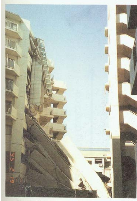
Overpass between buildings collapsed during Kobe earthquake of 1995
