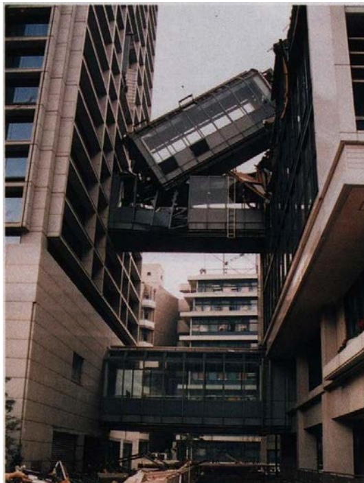
Overpass between buildings collapsed during Kobe earthquake of 1995
