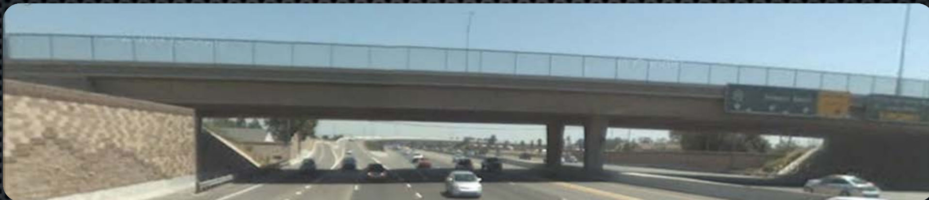
The La Veta Avenue Overcrossing
