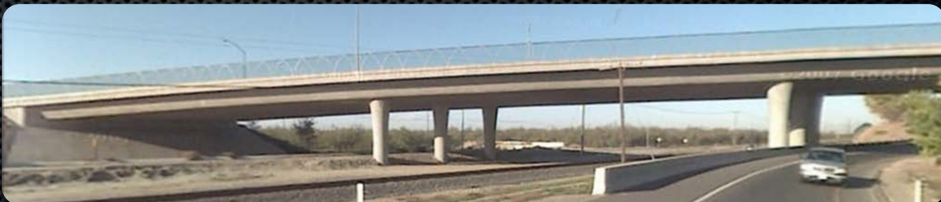
The Jack Tone Road Overhead
