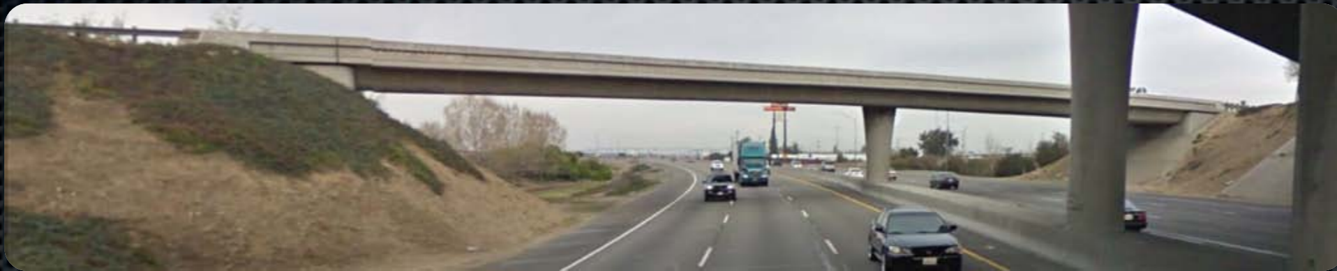
The Jack Tone Road On-Ramp Overcrossing
