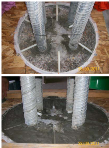
Shims and Mortar Bed between Column and Footing
