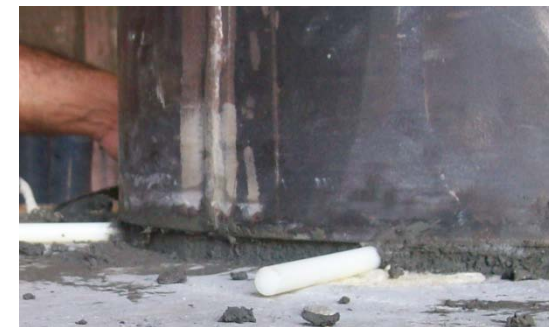
Metallic/Quartz Aggregate Mortar Bed Tooled to Ensure No Contact with External Shell
